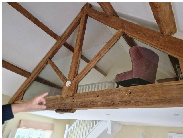
Internal photos to illustrate the creation of the mezzanine floor above the kitchen and dining space
