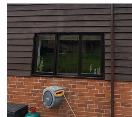
Existing kitchen timber window
