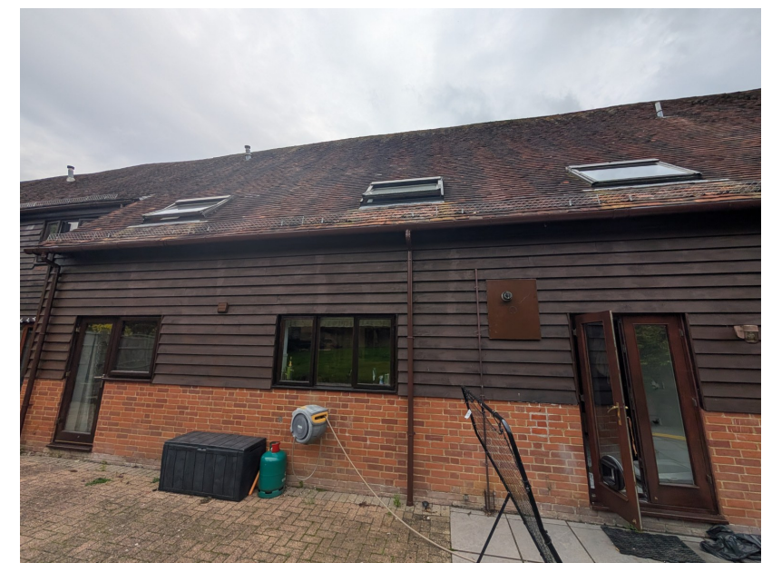
Existing window to rear.
