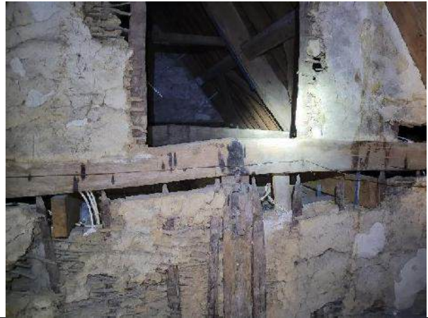
Photograph 14. Contiguous roof voids in Hazelbury Manor House (void 2).
