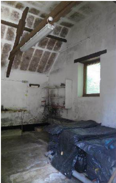
Photograph 43. B7, internal view of the converted stable into a storage area with a small roof void.
