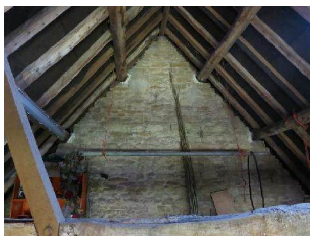
Photograph 30. B12 mezzanine floor and bitumen roof lining.
