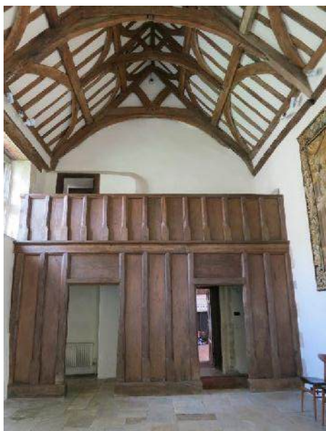
Photograph 11. Great Hall of Hazelbury Manor House with no roof void.
