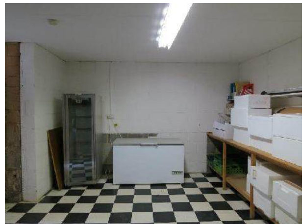
Photograph 36. Internal structure of B10 with breeze block and suspended ceiling.
