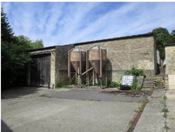
Photograph 35. B10 (Tythe Barn) with stone elevations and a corrugated sheet roof
