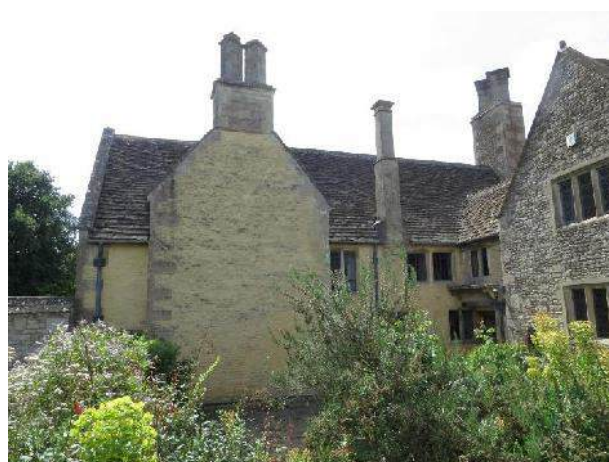
Photograph 10. Hazelbury Manor house
