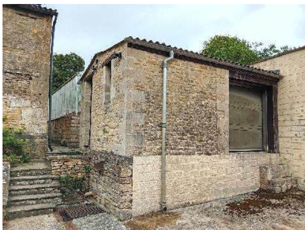
Photograph 39. B9 with a shallow pitched roof.
