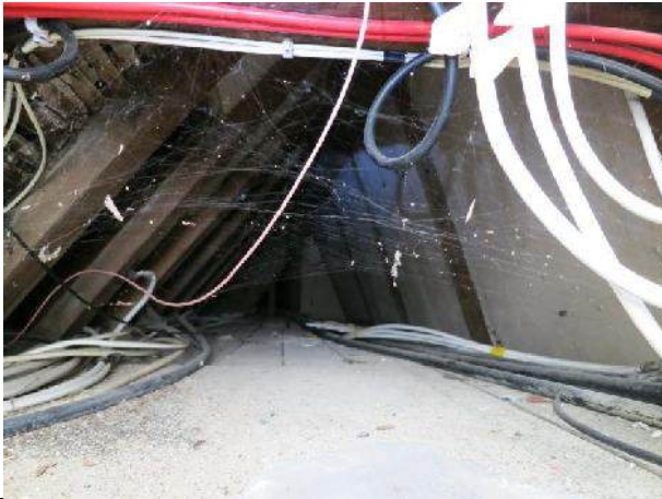
Photograph 13. Eaves cupboard / void in Hazelbury Manor House
