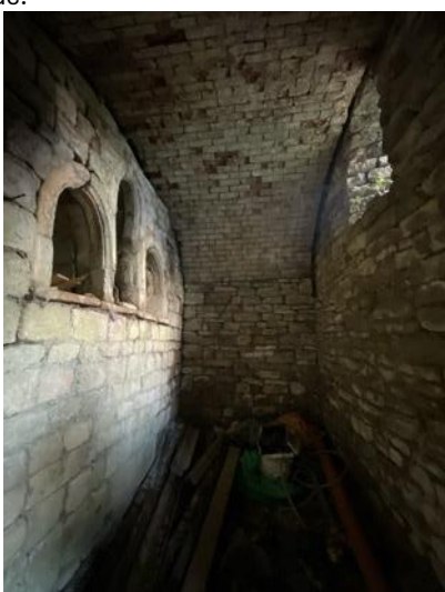
Photograph 15: Internal view of Chamber 2 room depicting internal windows through to Chamber 4.
