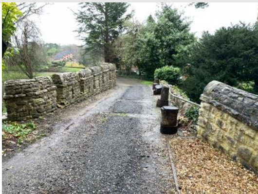
Photograph 1: Driveway over the Moat Bridge looking southeast (05/03/2024).
