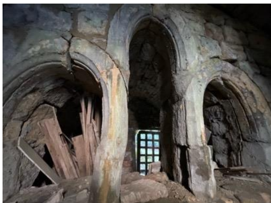
Photograph 17 View through from Chamber 2 to Chamber 4, depicting the latticed entrance gate.
