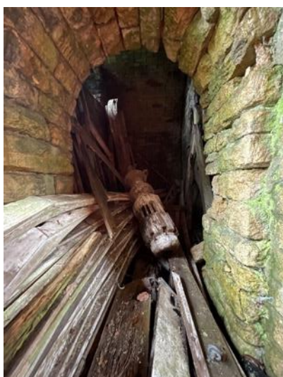
Photograph 19: Chamber 1 room on east elevation of the bridge, depicting storage of materials.
