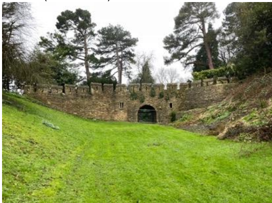
Photograph 3: East elevation viewed from the base of the moat.
