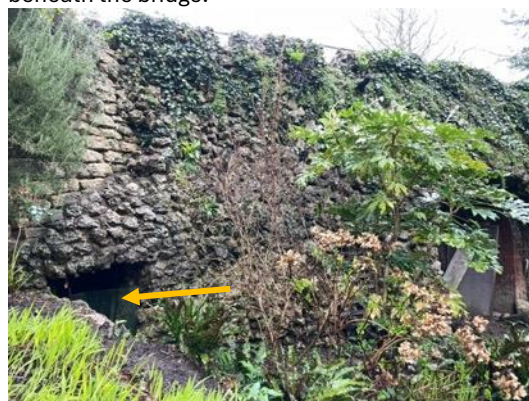
Photograph 8: Detail of entrance to Chamber 5 on west elevation.
