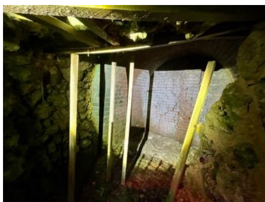
Photograph 10: Internal view of Chamber 5 at northern end of west elevation.
