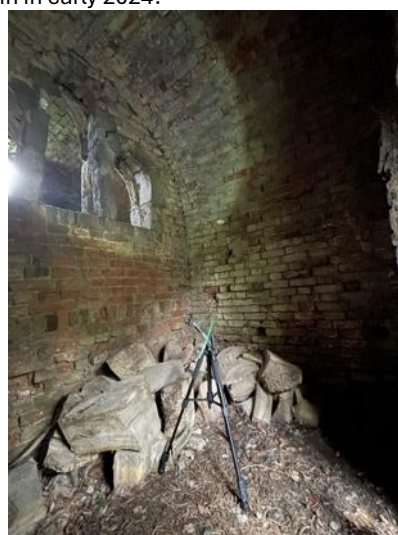
Photograph 20: Chamber 3 on the west elevation, depicting window through to Chamber 1 on the east elevation.
