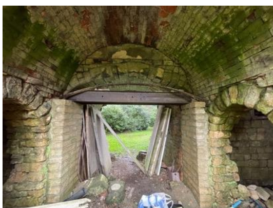
Photograph 13: Internal view of archway from the northeast, depicting doorways into Chambers 1 and 2 on either side.
