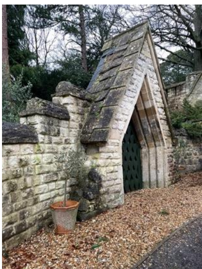
Photograph 5: Gate at northern end of Moat Bridge leading from the driveway down to the gardens owned by the neighbouring property.
