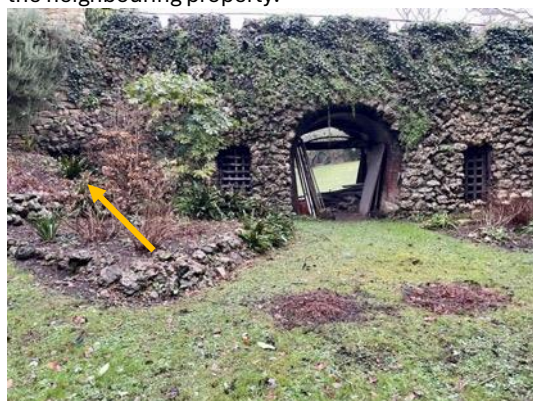
Photograph 7: Entrance to Chamber 5 on the west elevation visible at left of image.
