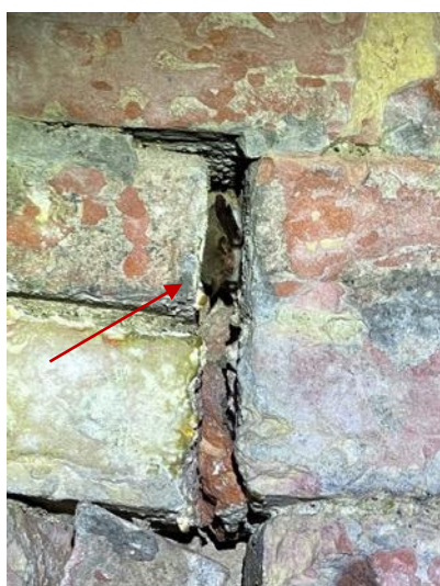
Photograph 21: Depicting Natterer's bat within the ceiling brickwork of Chamber 3.
