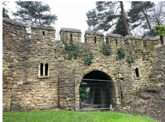
Photograph 4: Detailed view of the archway, depicting windows into Chambers 1 and 2 on the east elevation.
