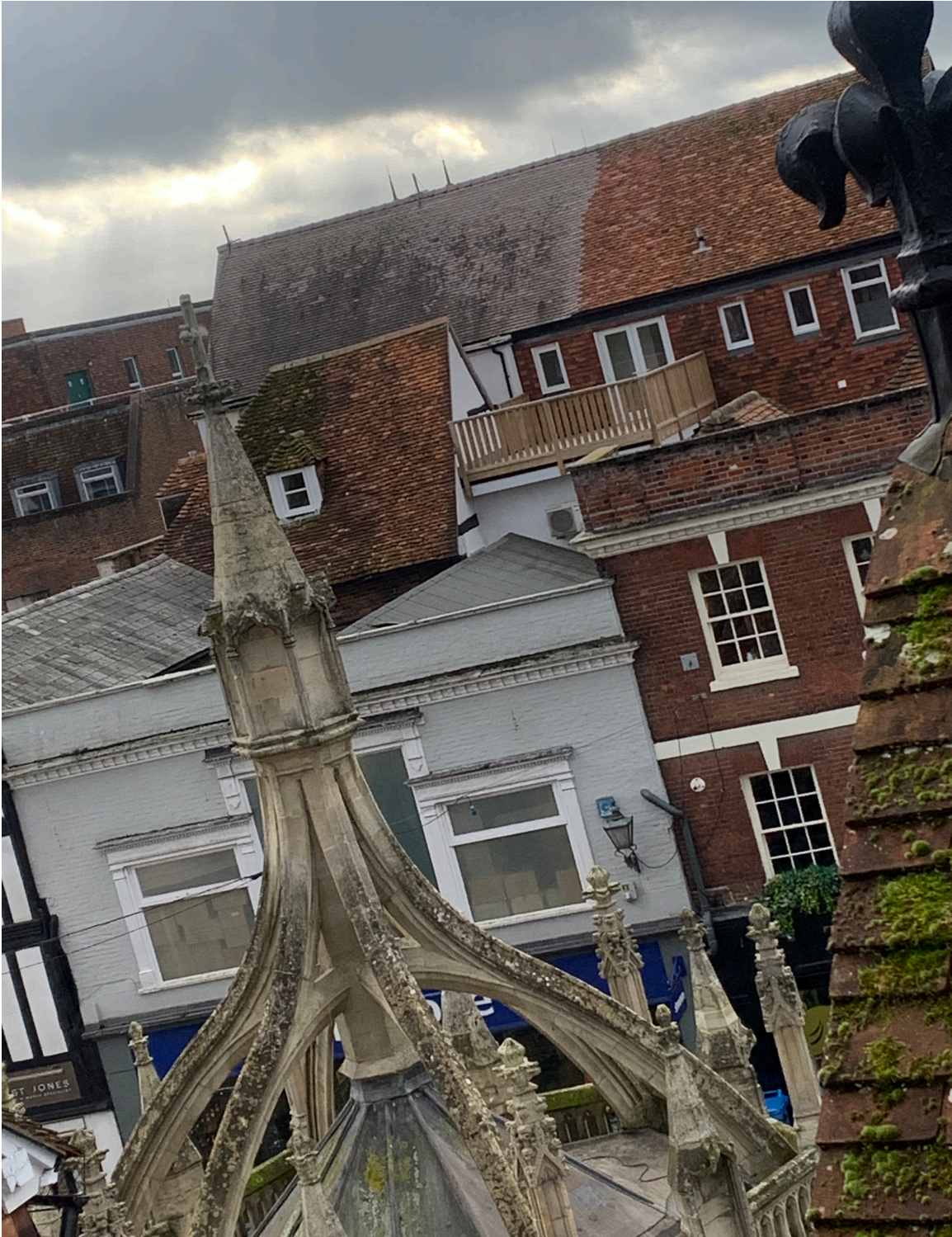
Photo 1 – Overhead view roof structure
