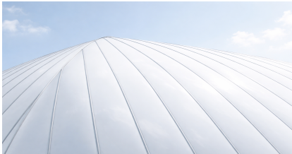
1. Air supported ETFE shell (translucent)
