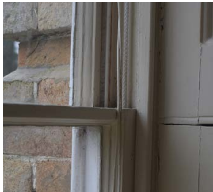
Window of the ground floor principal rooms are the earliest of the house, with fine glazing bars and meeting rails
