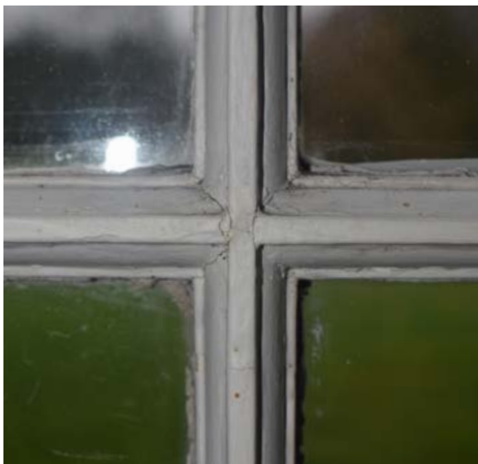
The late nineteenth century Frank Verity windows are focussed to the side and rear ranges and have clearly identifiable horn and glazing bar profiles
