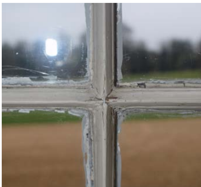
Window of the ground floor principal rooms are the earliest of the house, with fine glazing bars and meeting rails
