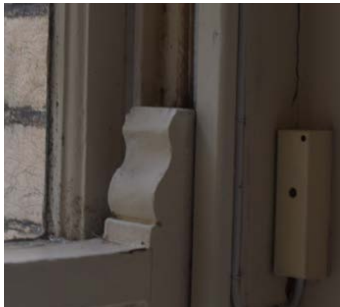
Frank Verity's substantial additions for Captain Freville Cookson are similar in design to both earlier phases of window but have horns to both upper and lower sashes
