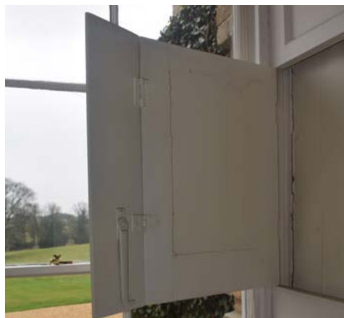
Window of the ground floor principal rooms are the earliest of the house, with fine glazing bars and meeting rails
