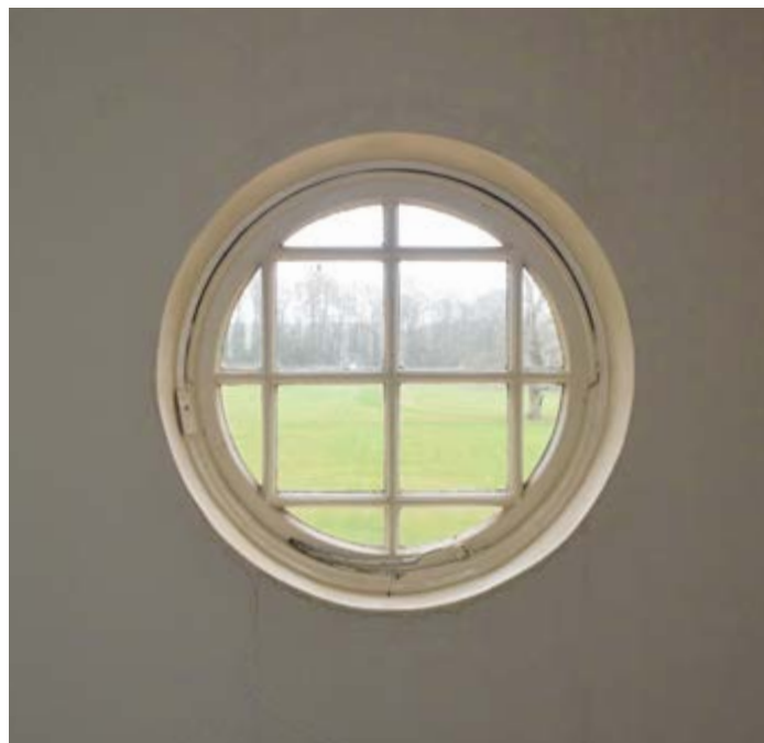
The late nineteenth century Frank Verity windows are focussed to the side and rear ranges and have clearly identifiable horn and glazing bar profiles
