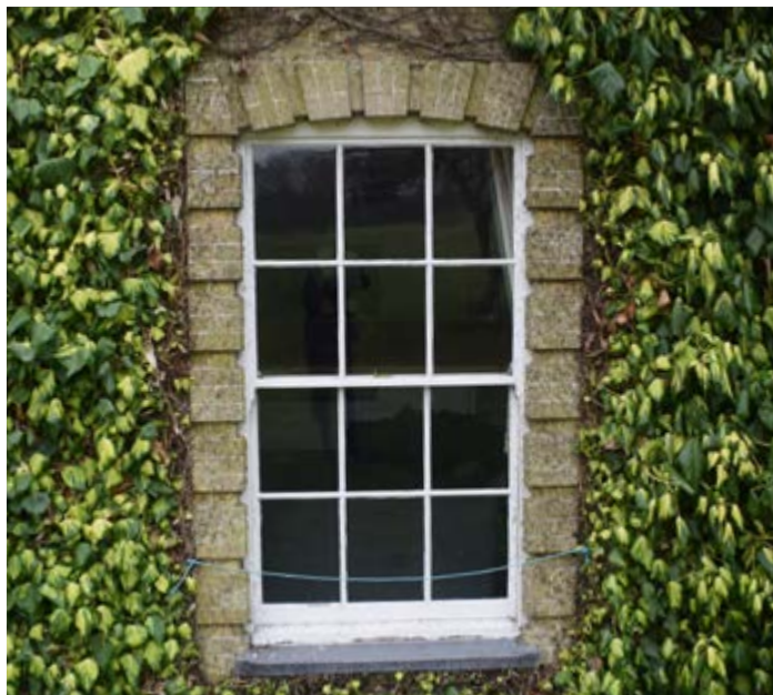
Frank Verity's substantial additions for Captain Freville Cookson are similar in design to both earlier phases of window but have horns to both upper and lower sashes
