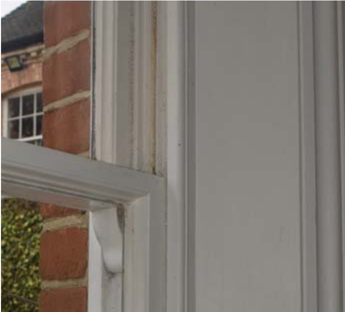
Horn detail of a late twentieth century sash window inserted post removal of the service range and later leaded lights within ground floor Verity casements
