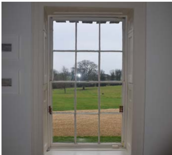
Window of the ground floor principal rooms are the earliest of the house, with fine glazing bars and meeting rails
