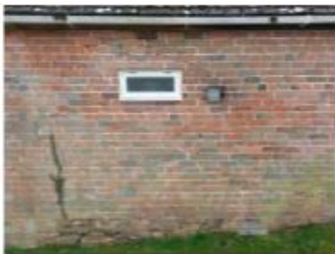
Window and Vent 2
