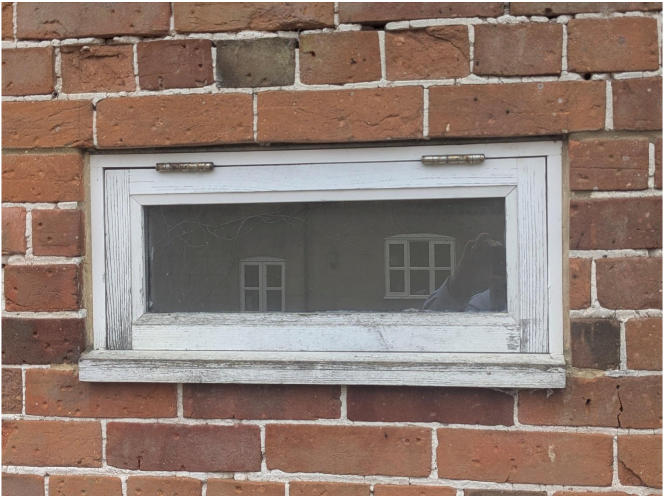
Window - installed Oct 2014
