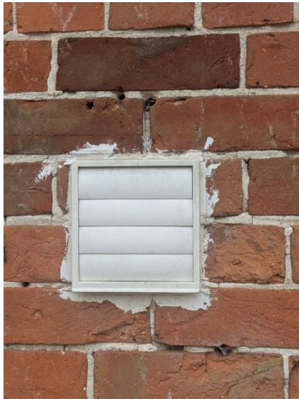
Vent 1 - installed Oct 2014
