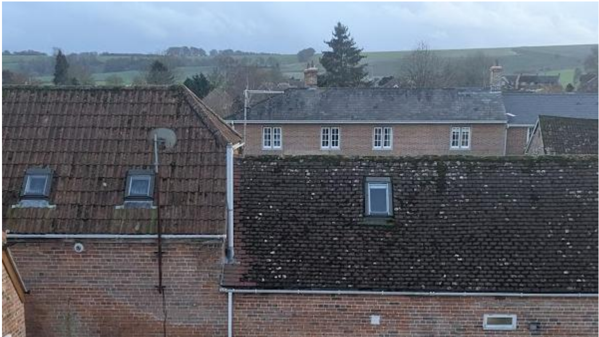
Roof lights x3, satellite dish, vents x 3, television aerial, new window
