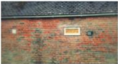
13 th October 2014 – window and vents installed
