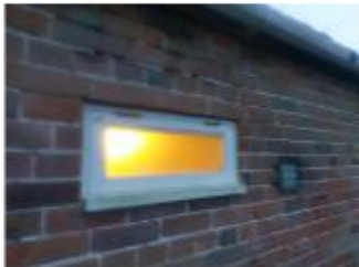
Window and Vent 2
