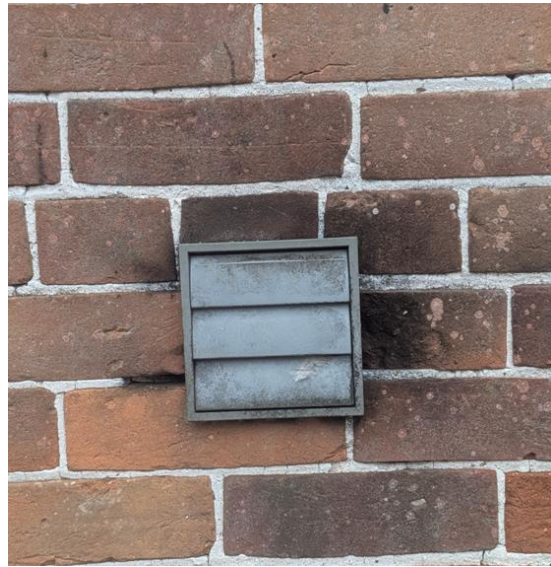
Vent 2 - installed Oct 2014
