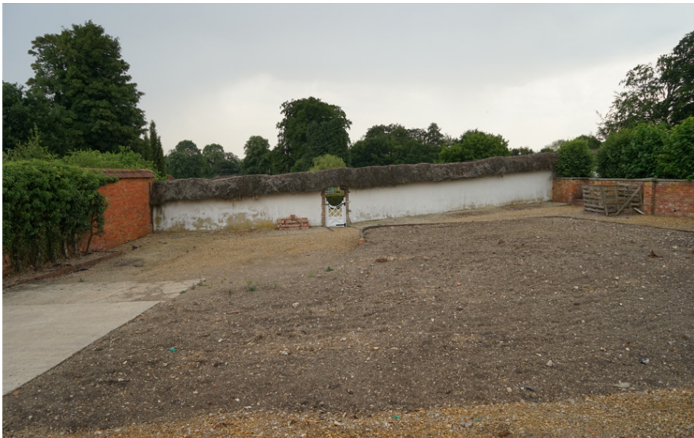
The southern side of the northern walled garden cobb with thatch wall
