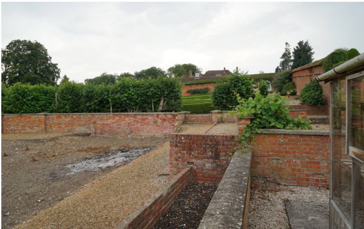
Looking west along the inside of the wall with the bases of the 1898 greenhouses and the house beyond
