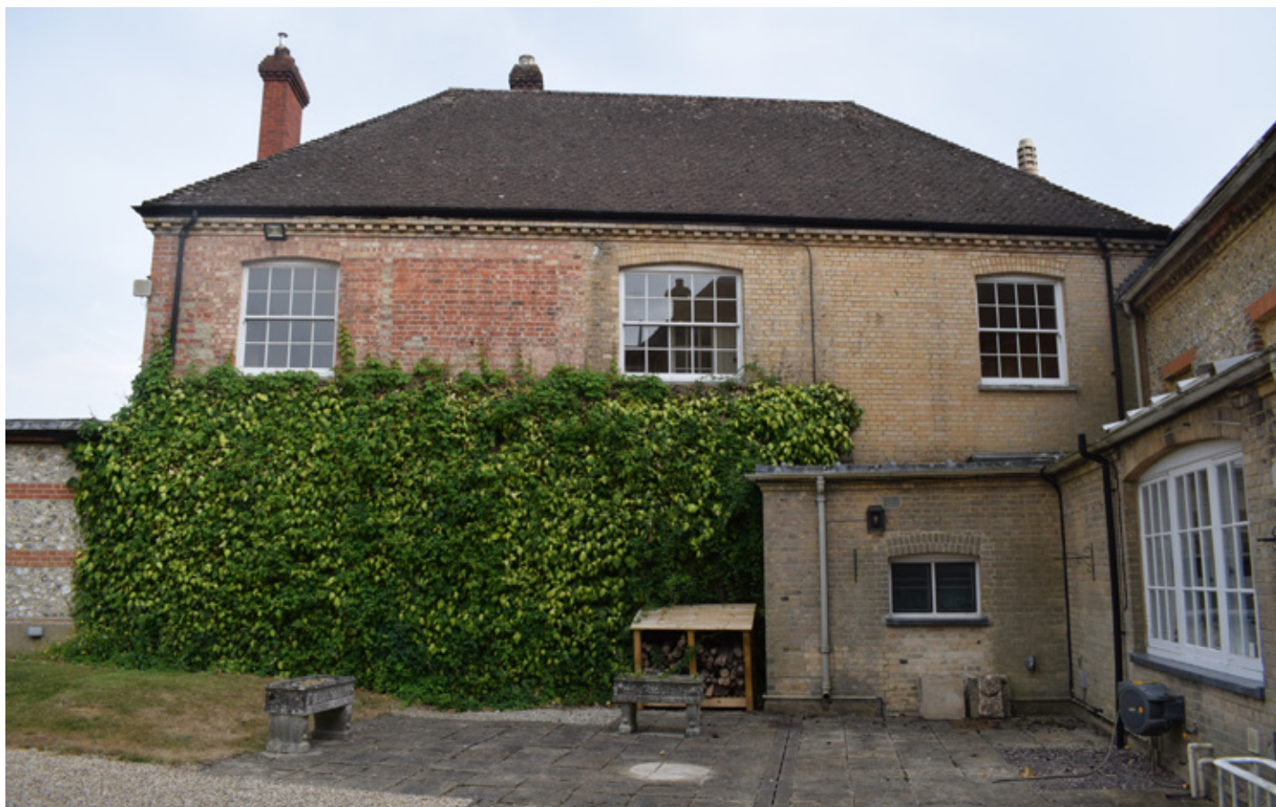
Rear (west) elevation of the coach house block. The brick infill evidence of it formerly linking to another 1897/8 wing, demolished c1986/7. Mixture of grey-buff and red bricks
