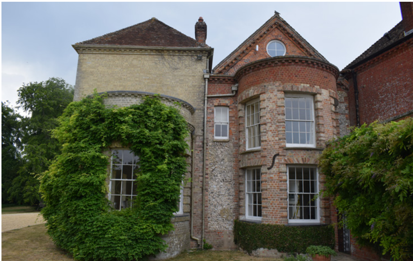
The east end elevation with the gabled flint and brick late 17th century range with the 18th bay, and the c1750 hipped and grey-buff brick range to the south, and the end wall of the 1897/8 coach house
