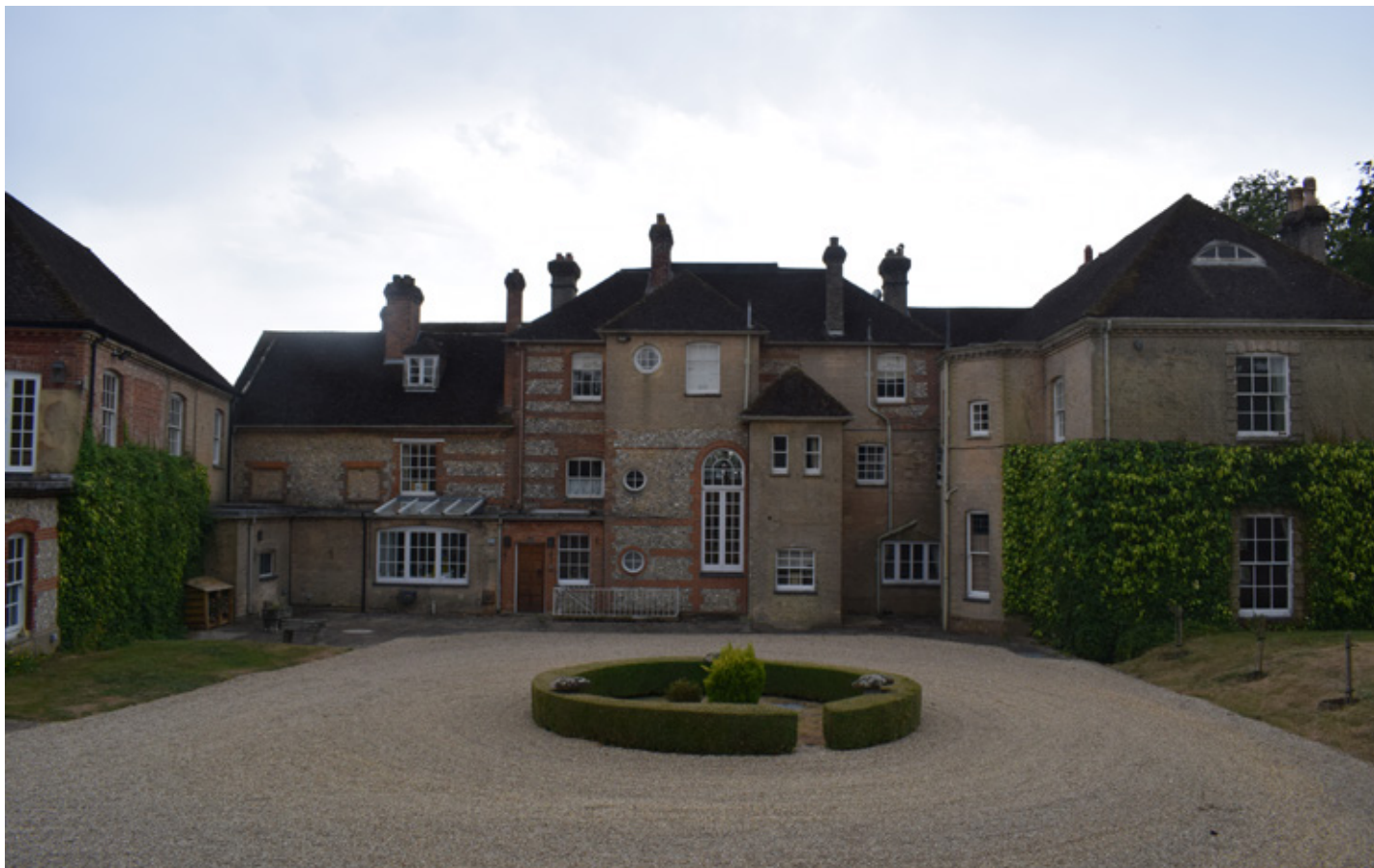
The rear (north) elevation of the house following the removal of the 1897/8 additions in 1986/7. The surviving earlier two-storey range with flint and brick lies to the left-hand side, with the 1897/8 coach house range
