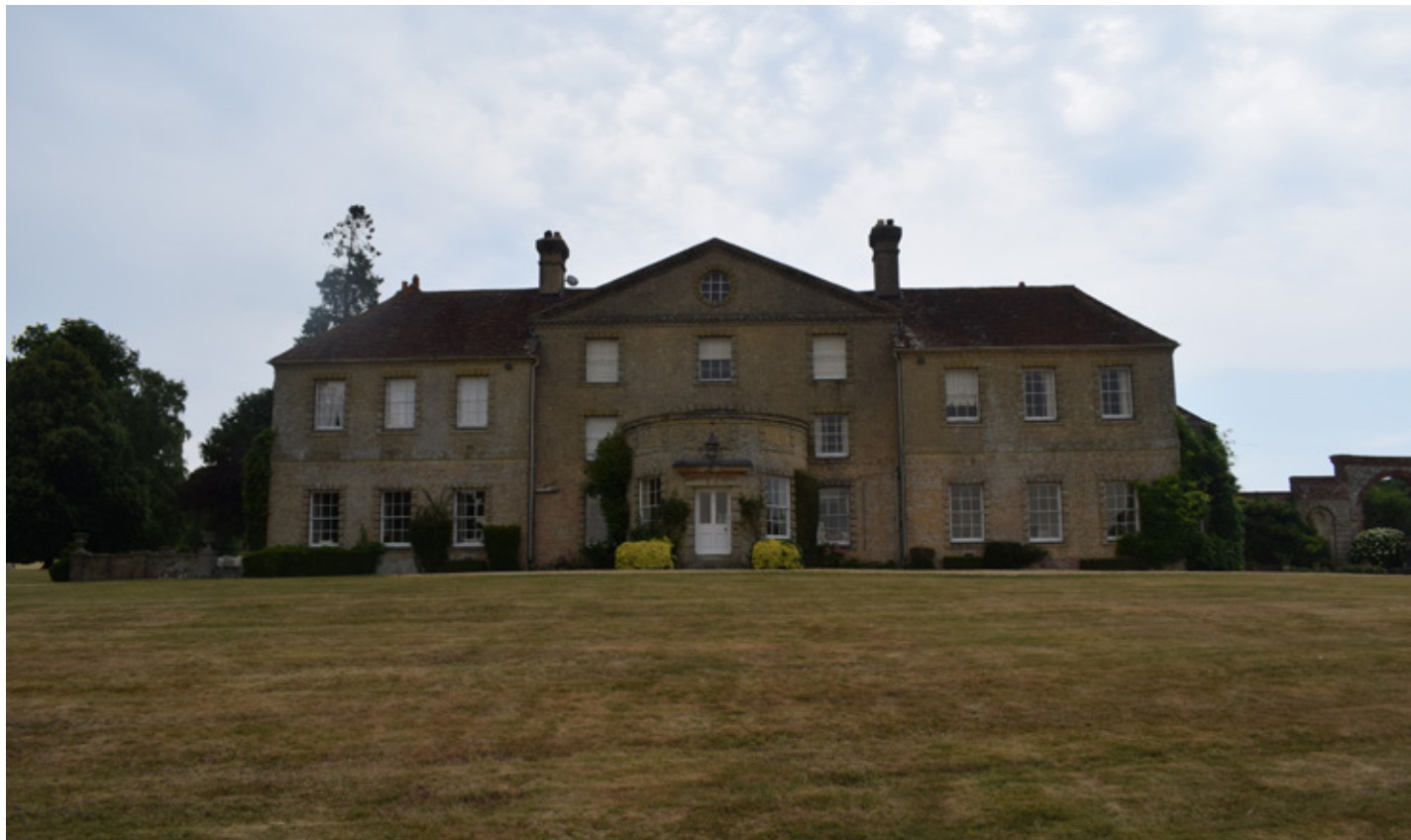
The principal front (south) elevation of the house, c1750 by James Pulse, with later circular porch, added to an earlier 17th range to the north
