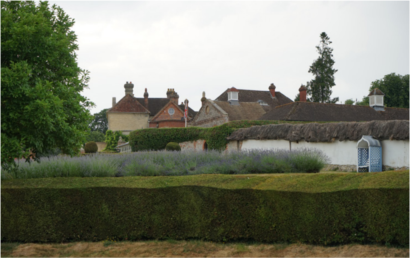
View of the cobb and thatched wall looking towards to service yard and house provide a picturesque composition
