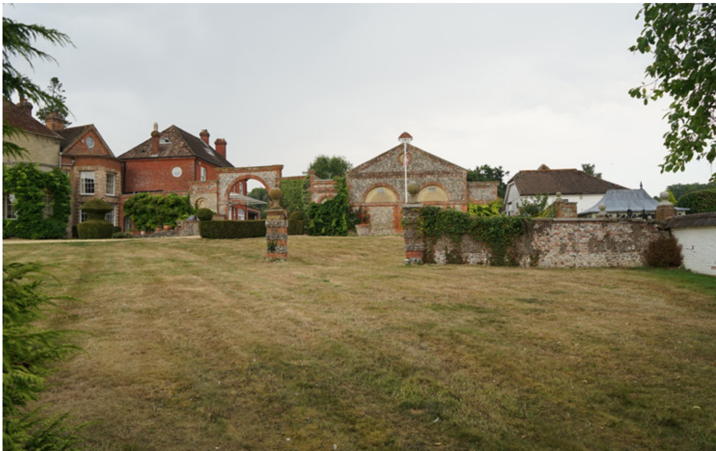
View of the service yard, stables from the south , the gate piers showing the location of the earlier drive to the yard
