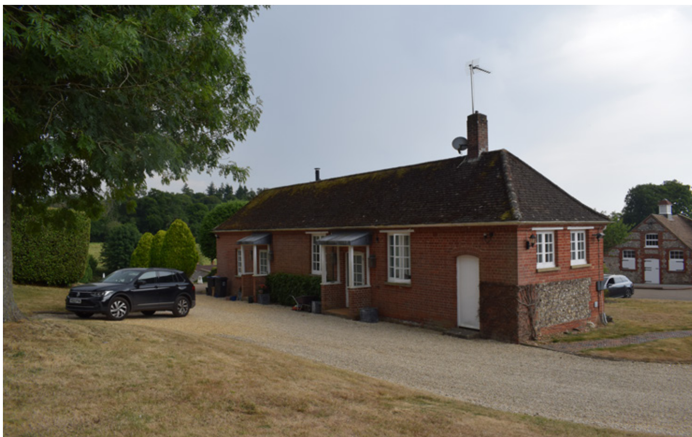
The north elevation of the 1977 bungalow
