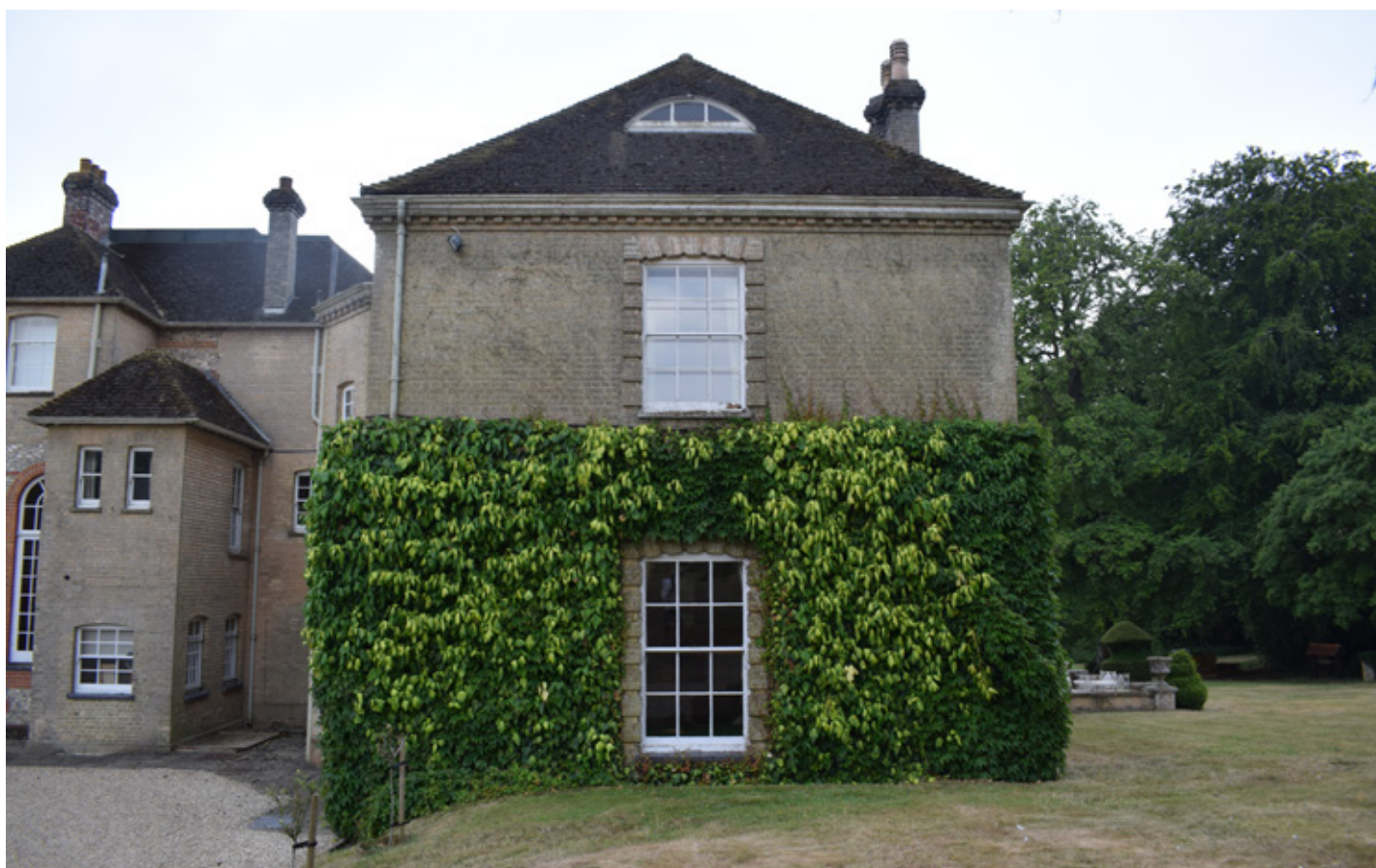
The northern end of the 1897/8 western wing
