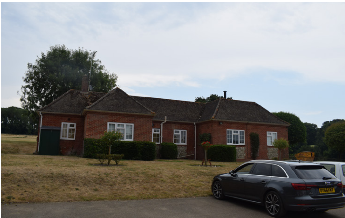
South elevation of the 1977 bungalow
