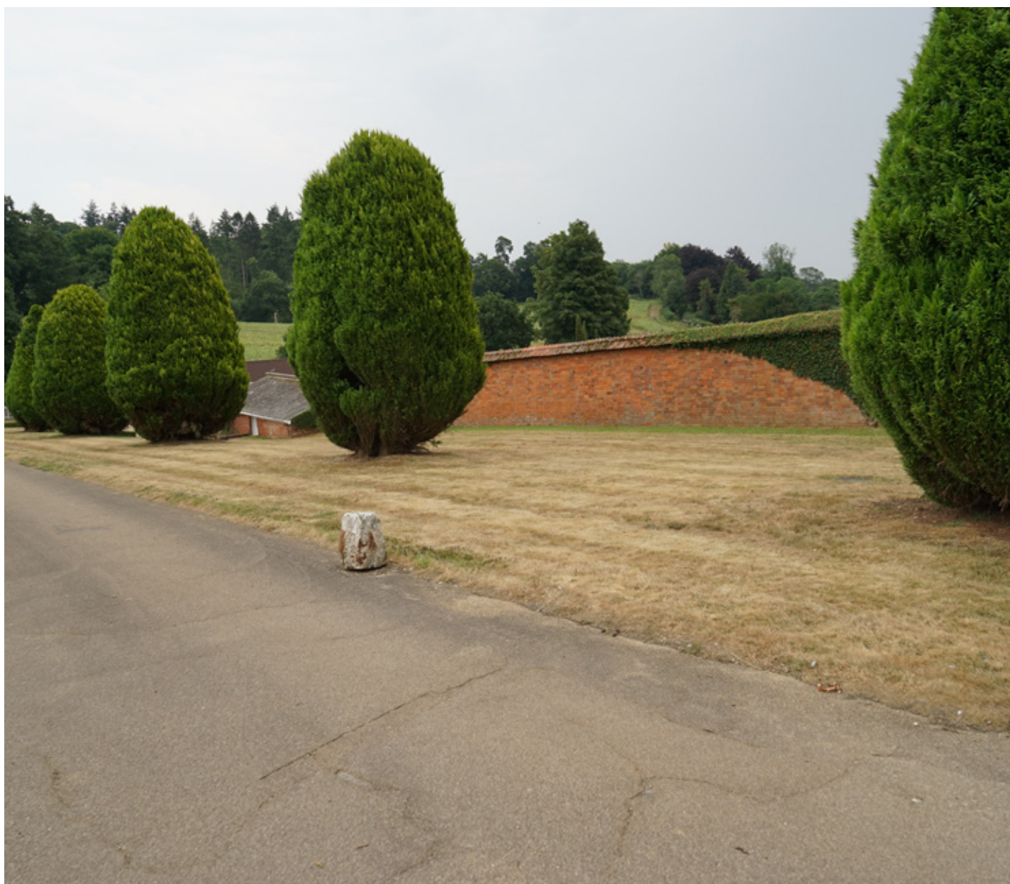
Northern wall of post 1897 garden looking east with roof of the former boiler house for the 1898 hot houses (greenhouses) on the inside of the wall since demolished
