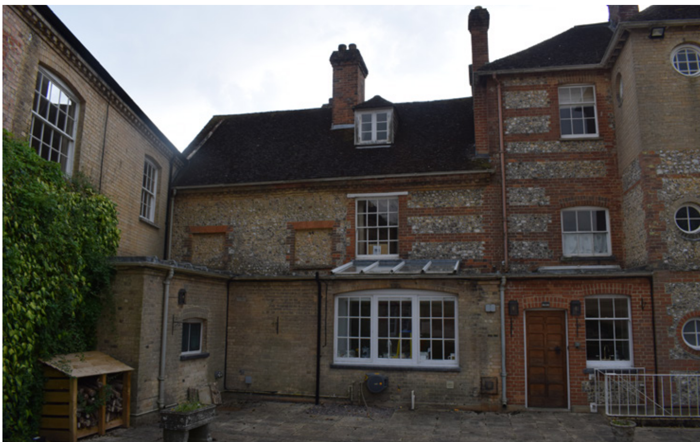
Portion of the late 17th flint and brick wing with blocked windows
