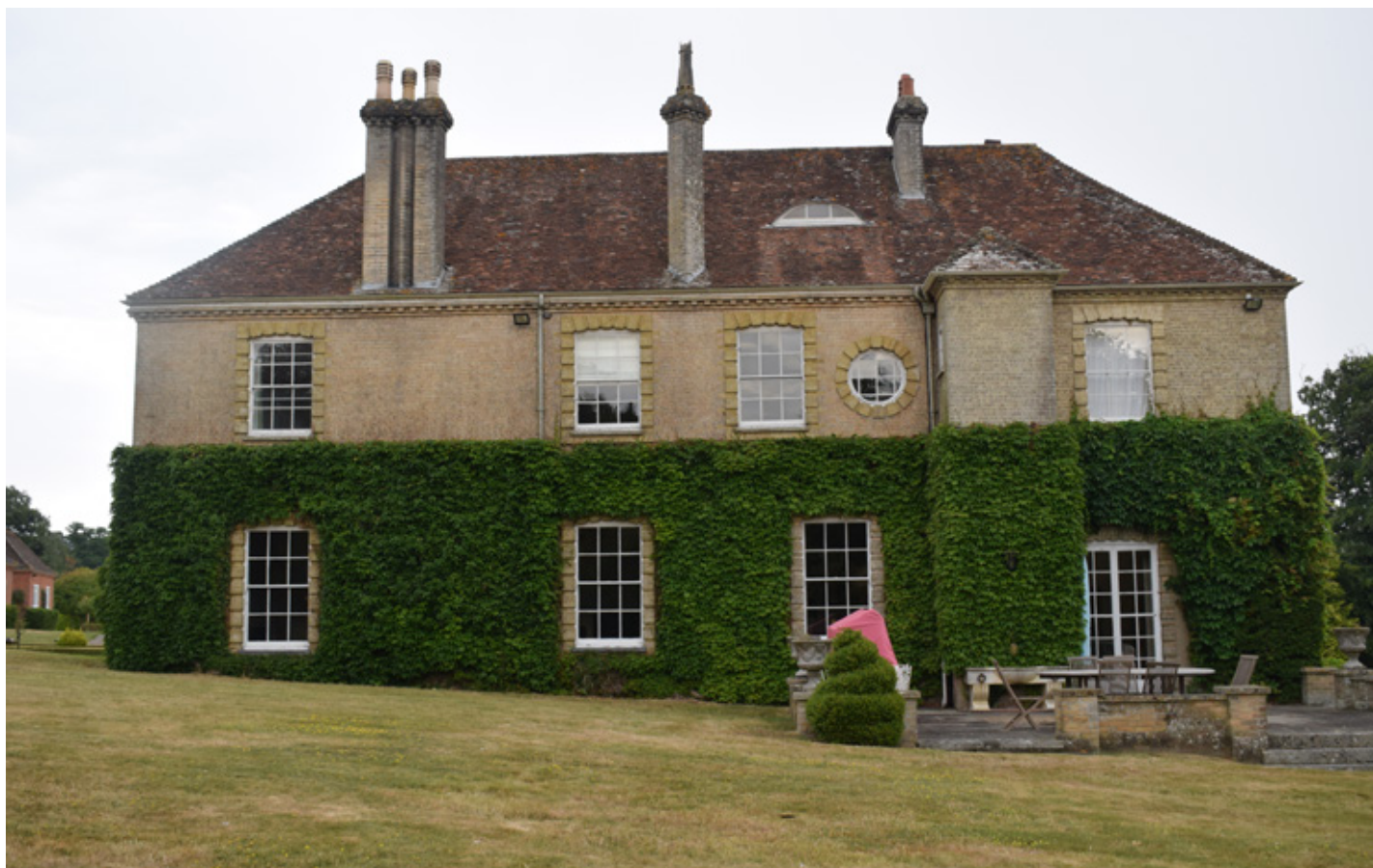
The west elevation of the c1750 house with the 1897/8 wing to the left-hand side of the two-storey projection, using the same grey-buff bricks
