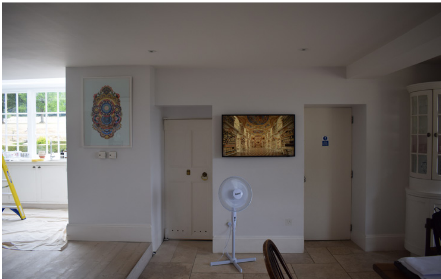
Northern side of Breakfast room silver safe and storeroom
