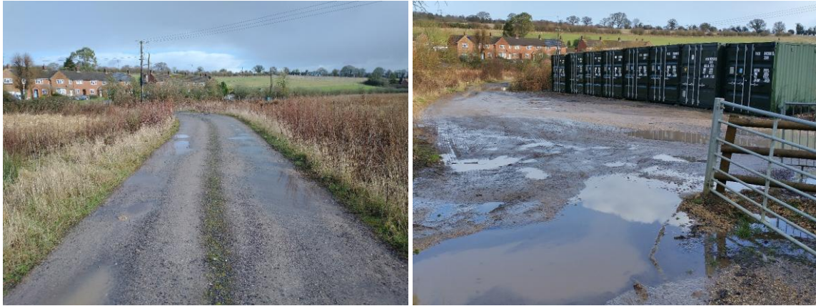
Figures 1 and 2: Access track and gravel area in east of site, respectively.
