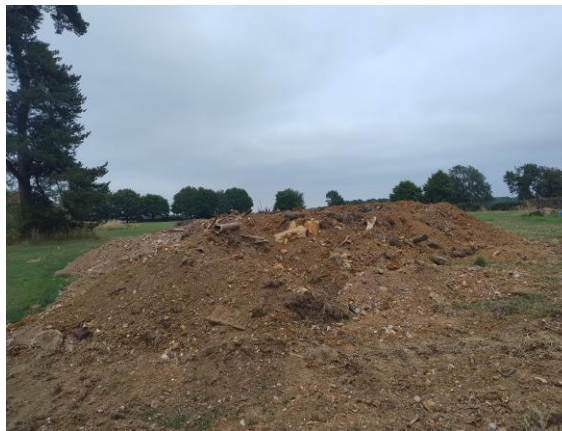
Figure 2: Spoil heap present due to current works
