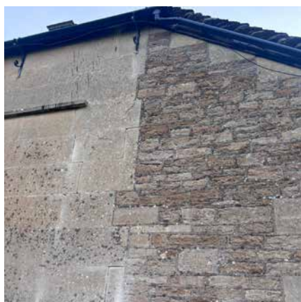
Rear elevation - junction in stonework
