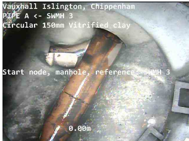
PIPE AX_105ae49c-3665-475b-8c64-7f1c6f9a6733_20230711_090 105_072.jpg, 00:00:00, 0.00 m Start node, manhole, reference: SWMH 3
