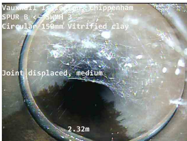
SPUR BX_c587a638-227b-4f95-9bcc-3111752f9d1c_20230711_092 052_683.jpg, 00:00:52, 2.32 m Joint displaced, medium
