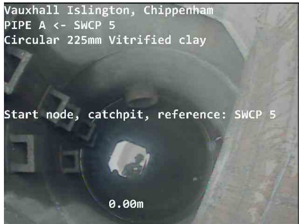
PIPE AX_50b7f84e-543b-4ef7-8b8a-f32d1a3acdf6_20230711_0958 08_911.jpg, 00:00:08, 0.00 m Start node, catchpit, reference: SWCP 5
