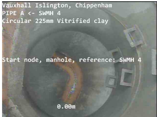
PIPE AX_a3d10040-91b9-4e4c-a50c-d5602dfb9778_20230711_09 3438_730.jpg, 00:00:00, 0.00 m Start node, manhole, reference: SWMH 4
