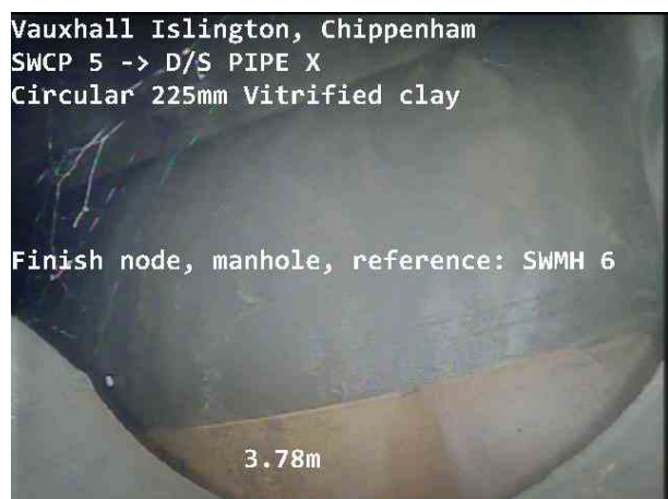
SWCP 5X_a5a0e31d-4632-4ecd-a1fd-1a1627f9144e_20230711_100 418_850.jpg, 00:00:41, 3.78 m Finish node, manhole, reference: SWMH 6
