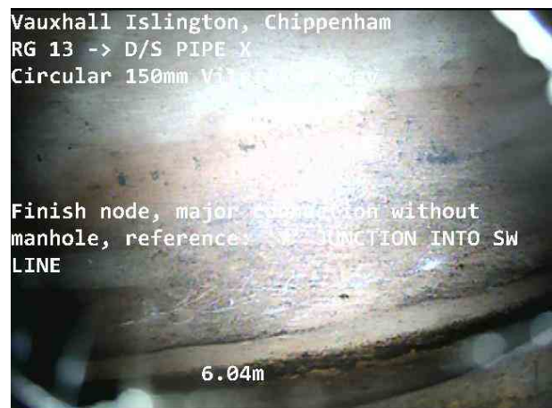
RG 13X_bc63ce0e-a2eb-4454-acbe-d1c81d1f748b_20230711_13 3718_094.jpg, 00:01:21, 6.04 m Finish node, major connection without manhole, reference: 'Y' JUNCTION INTO SW LINE
