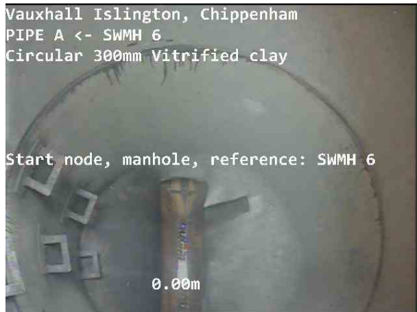
PIPE AX_18f06710-722a-4d24-a1fb-e13d92f66312_20230711_101 523_127.jpg, 00:00:00, 0.00 m Start node, manhole, reference: SWMH 6
