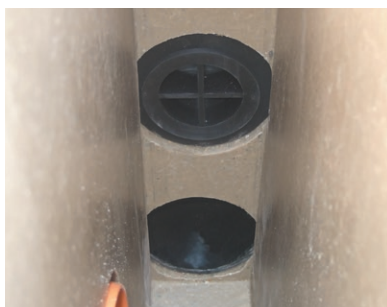
View of foul air trap before installation
