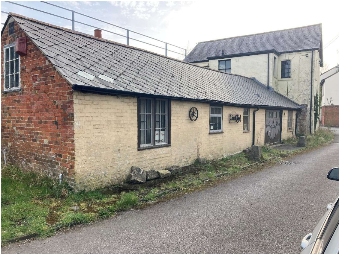
View of the Canal Forge looking towards the south-west.
