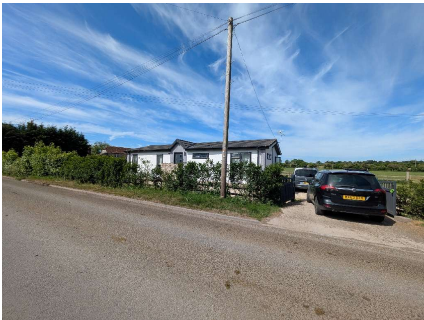
Existing front elevation and driveway / highway access
