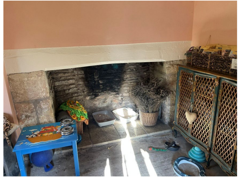
Plate 20: Open fireplace with stone lintel and jambs
