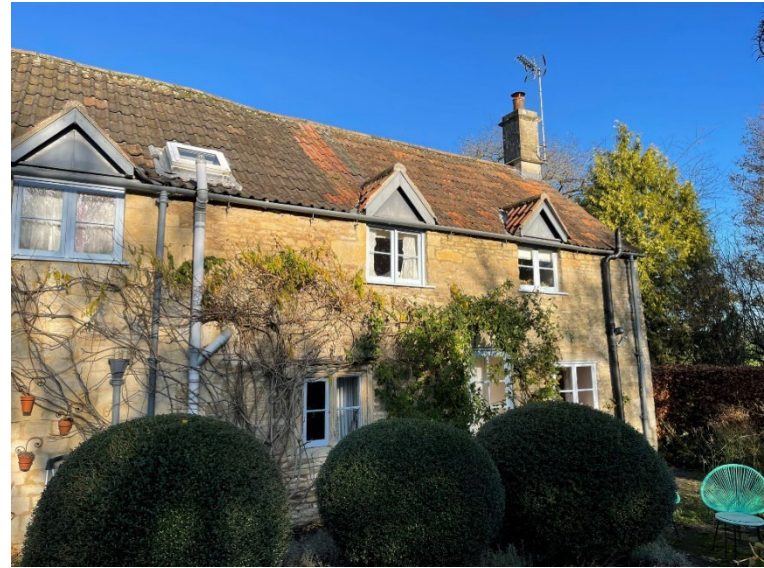
Plate 10: Right side of south elevation
