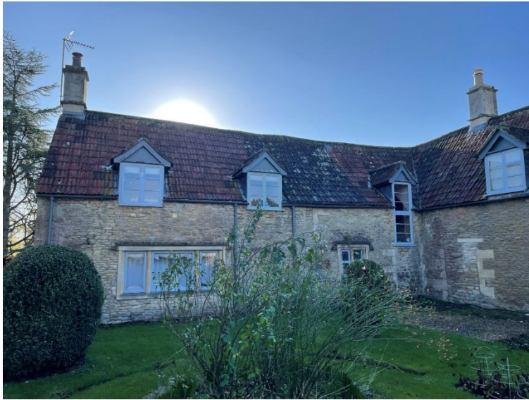
Plate 15: North elevation with 20 th -century ground floor window which replaced a garage door opening
