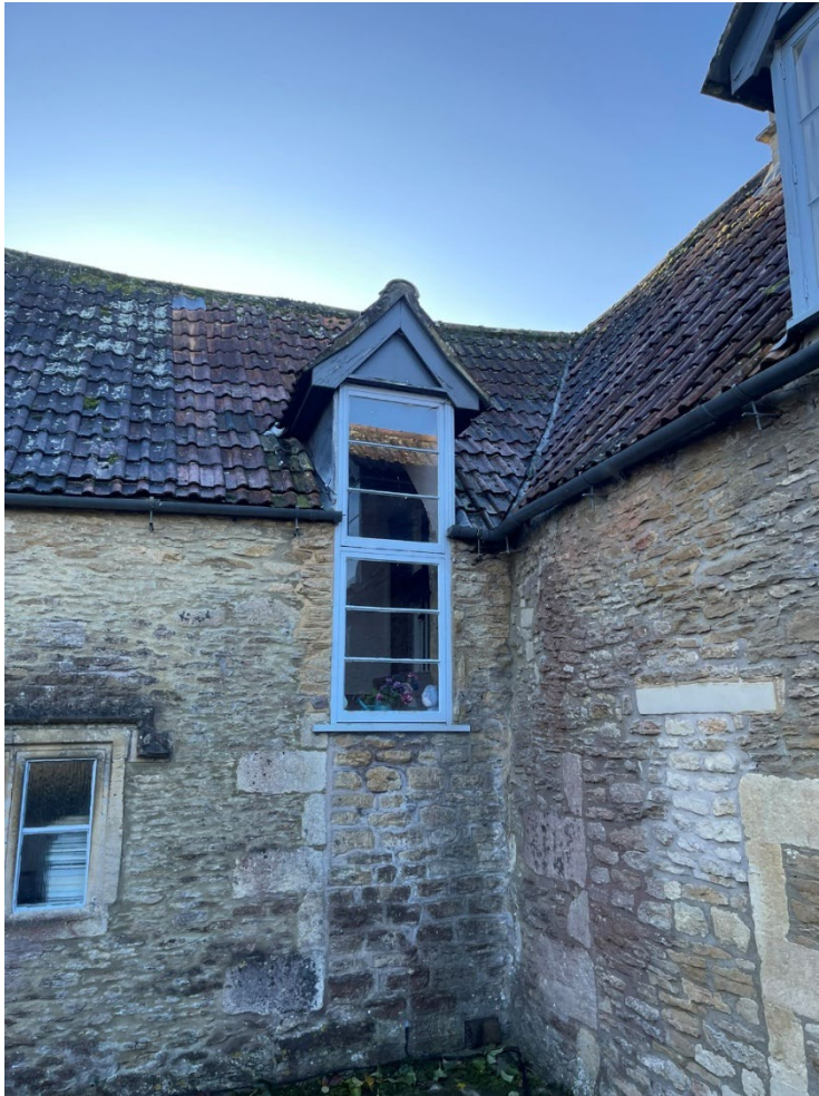
Plate 13: Close up view of the junction between earlier cottages and 19 th -century north cottage
