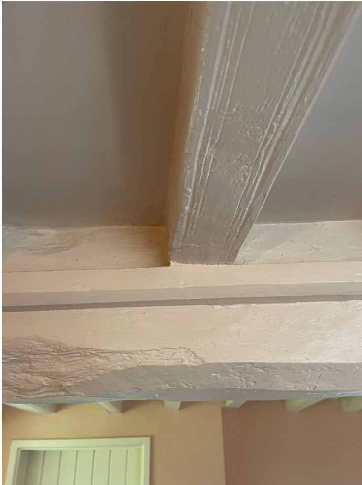
Plate 21: Chamfered ceiling beams and later grooved joists
