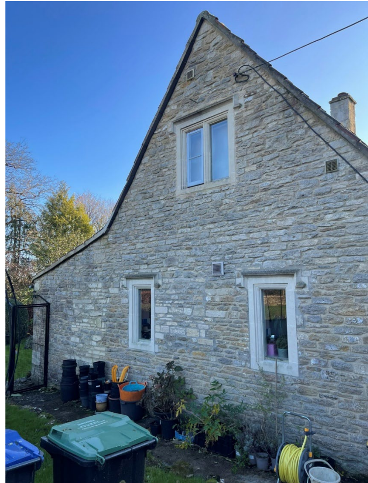
Plate 18: North gable end of 20 th century north wing
