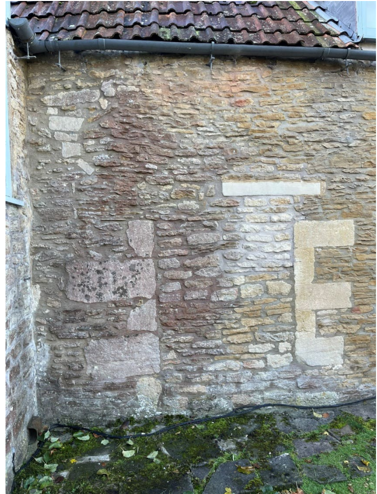
Plate 14: Blocked doorway with quoins to north cottage
