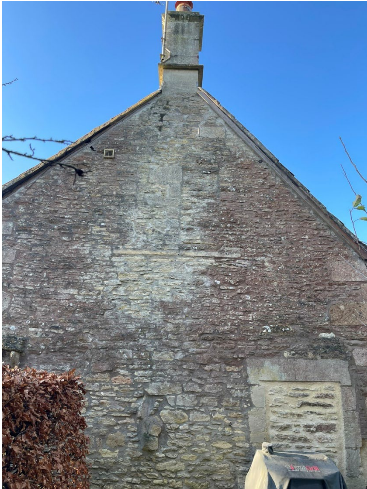
Plate 11: Blocked openings on east gable end
