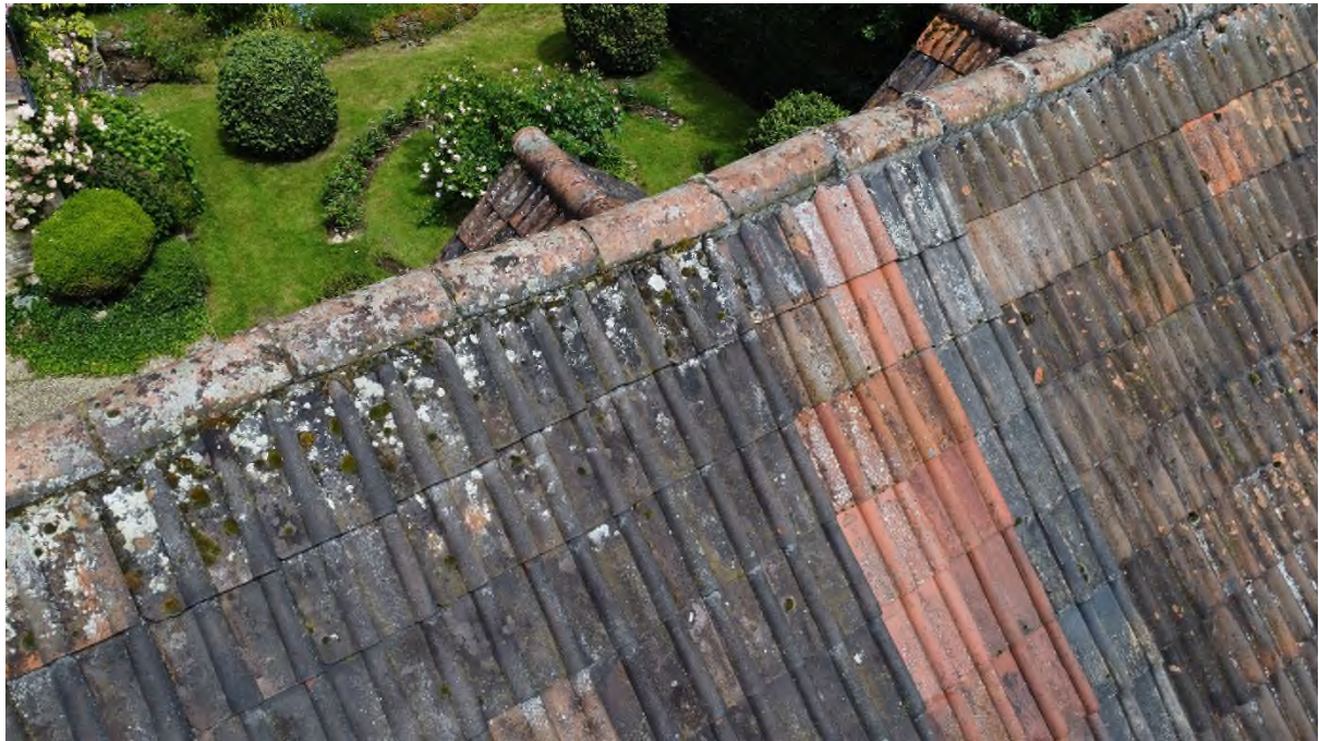
Plate 3 Roof ridge well maintained and no obvious entry points for birds or bats
