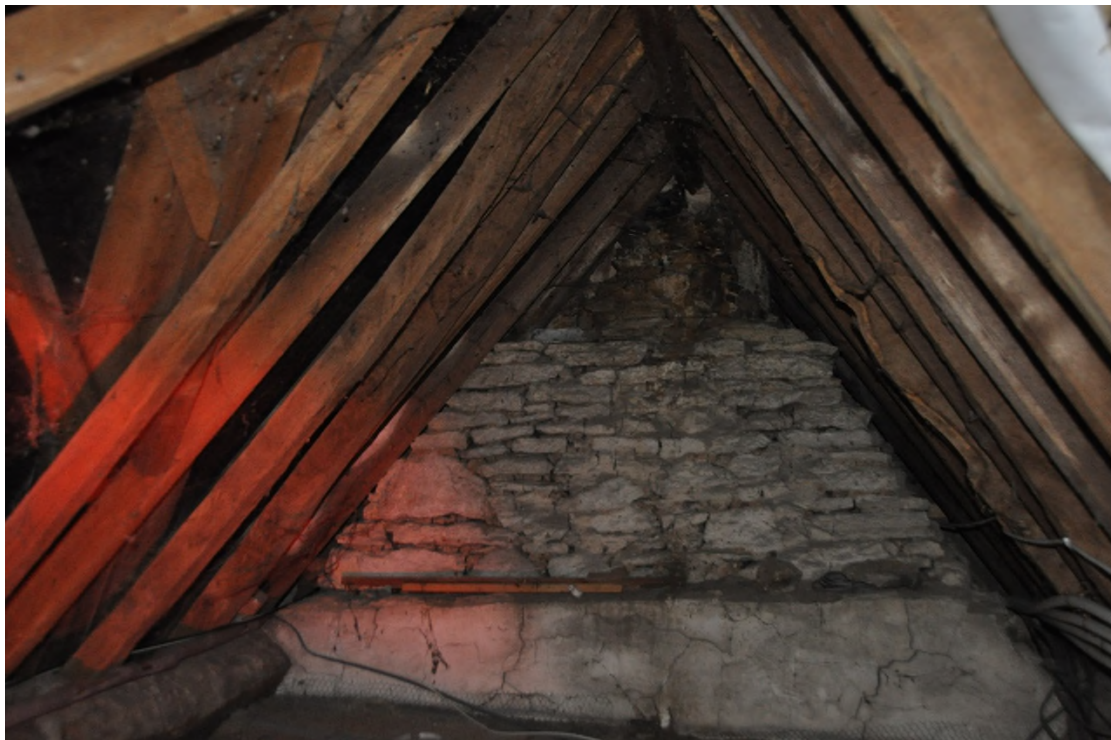
Plate 6 common rafter and purlin roof void throughout
