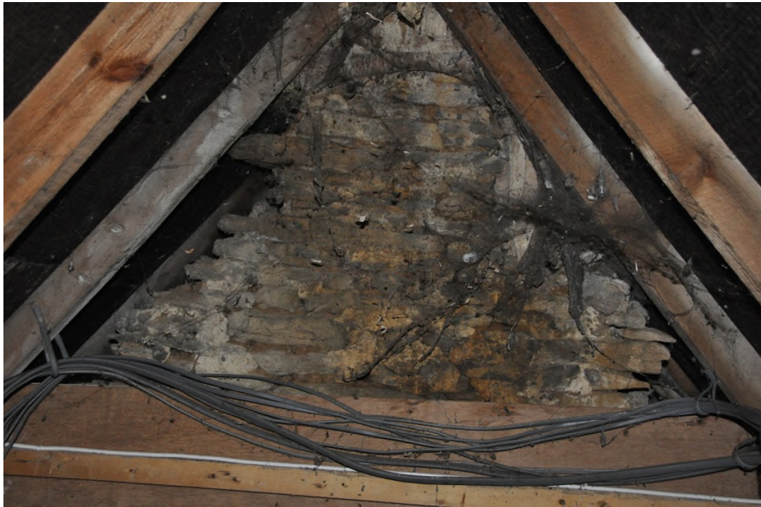
Plate 5 roof void filled with cobwebs showing no bats have been flying inside the void
