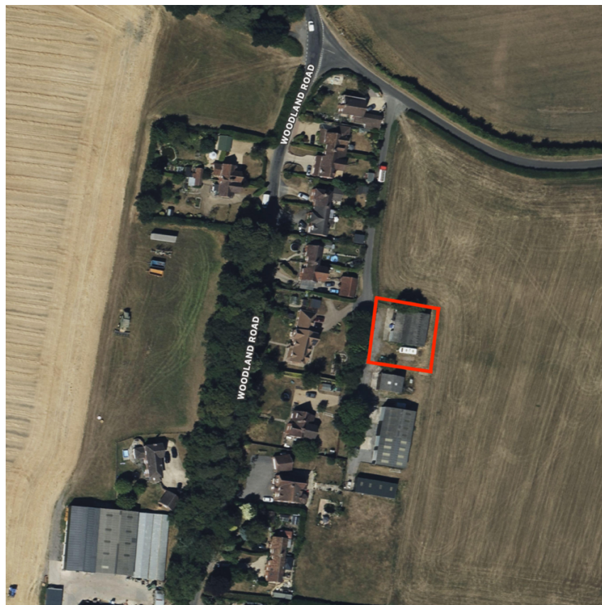
Figure 1: Satellite Photo showing the existing building
