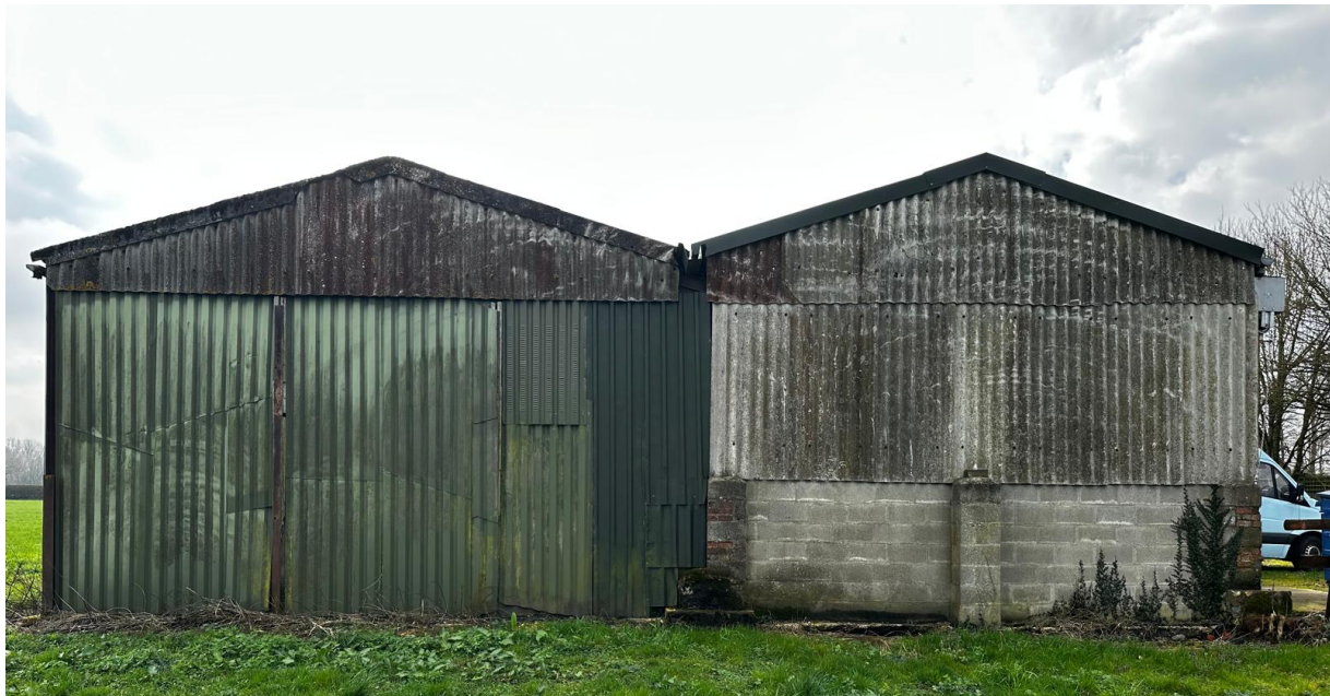
Figure 2: Photo of the Northern Elevation
