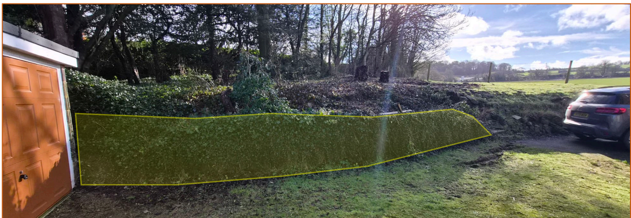
Image 1: A small section of the existing retaining wall (yellow annotation) will be replaced. The differences in ground levels mean that a root bridging system is not possible in this situation
