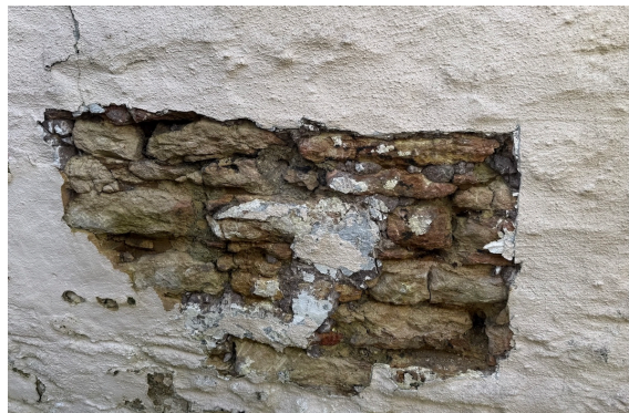
Section of wall with render removed to expose random stone
