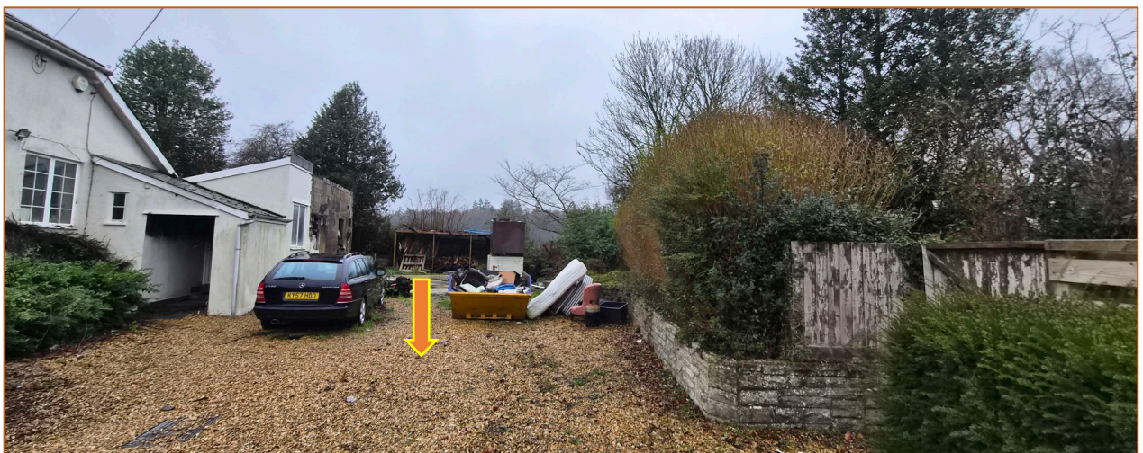
Image 2: Materials can also be delivered to site using the existing access and there is plenty of space to store and move them to the working areas
