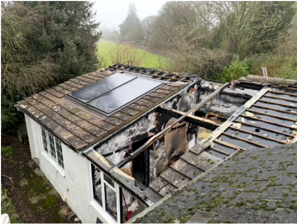
Figure 8. Interior of fire-damaged wing
