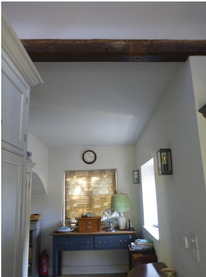
Fig 7: There is an inaccessible loft space above the smaller extension that will be affected by the new extension proposals for Stop Farm.
