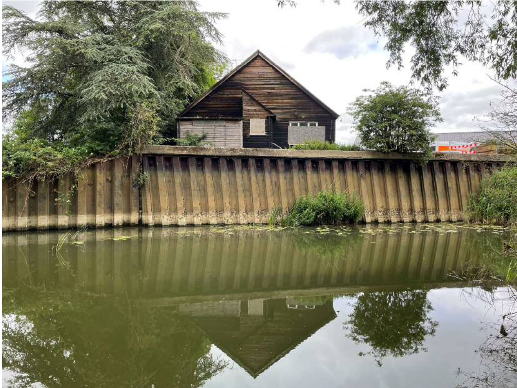
Photograph 5: View across the River Avon towards the north of the sheet pile wall and timber clad former gym/scout hut in the southwest of the site.
