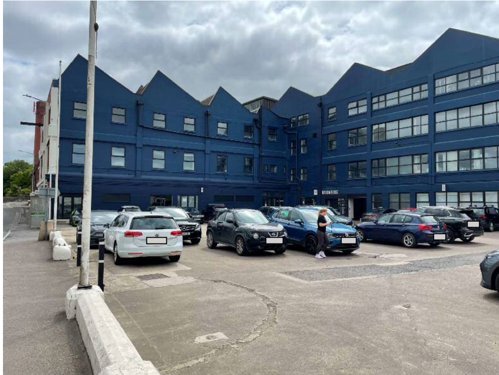
Photograph 1: View south east of the main site frontage (Units A, B, D to F).
