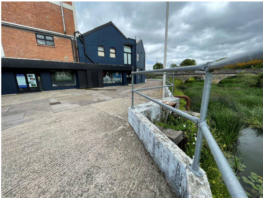
Photograph 6: View east of Units C and G, top of the concrete retaining wall adjoining the River Avon and the sluice structure.
