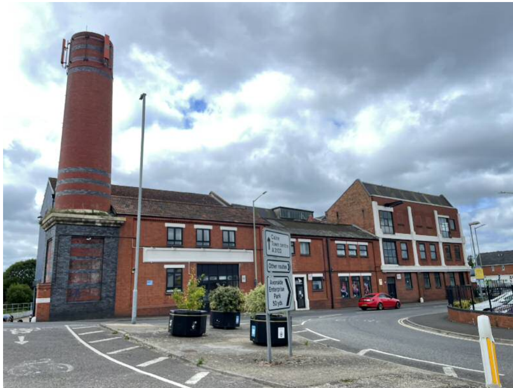
Photograph 2: View south from New Broughton Road of Units D to F.
