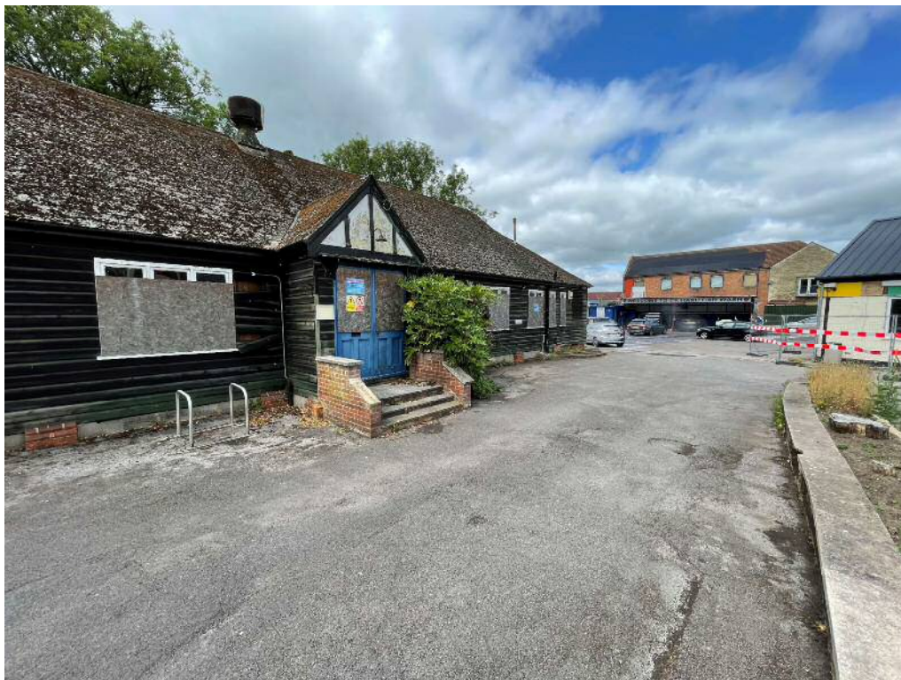
Photograph 8: View towards the northwest of the former gym/scout hut and the hand car wash.
