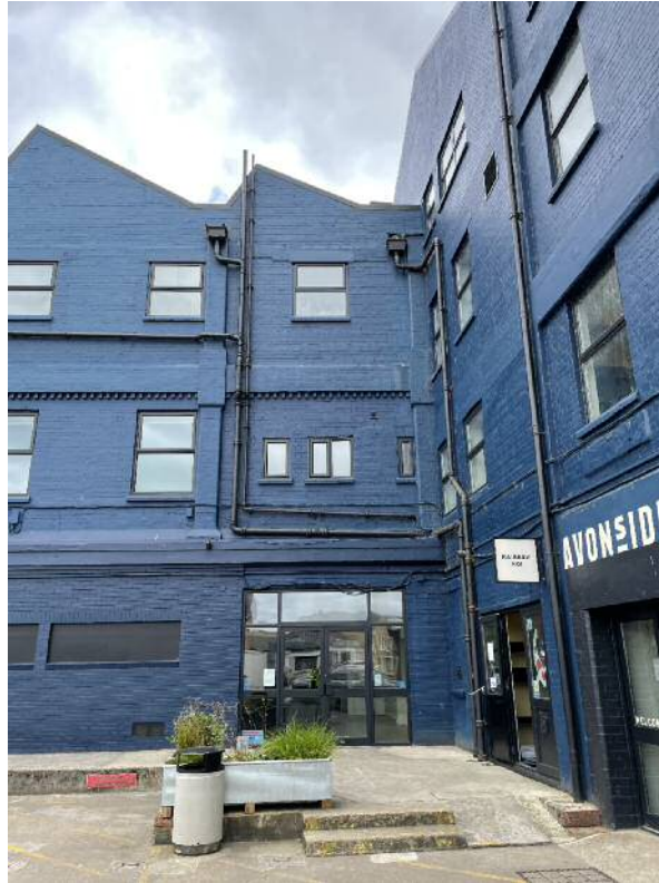
Photograph 11: View towards the east of the section of Unit D proposed for demolition.
