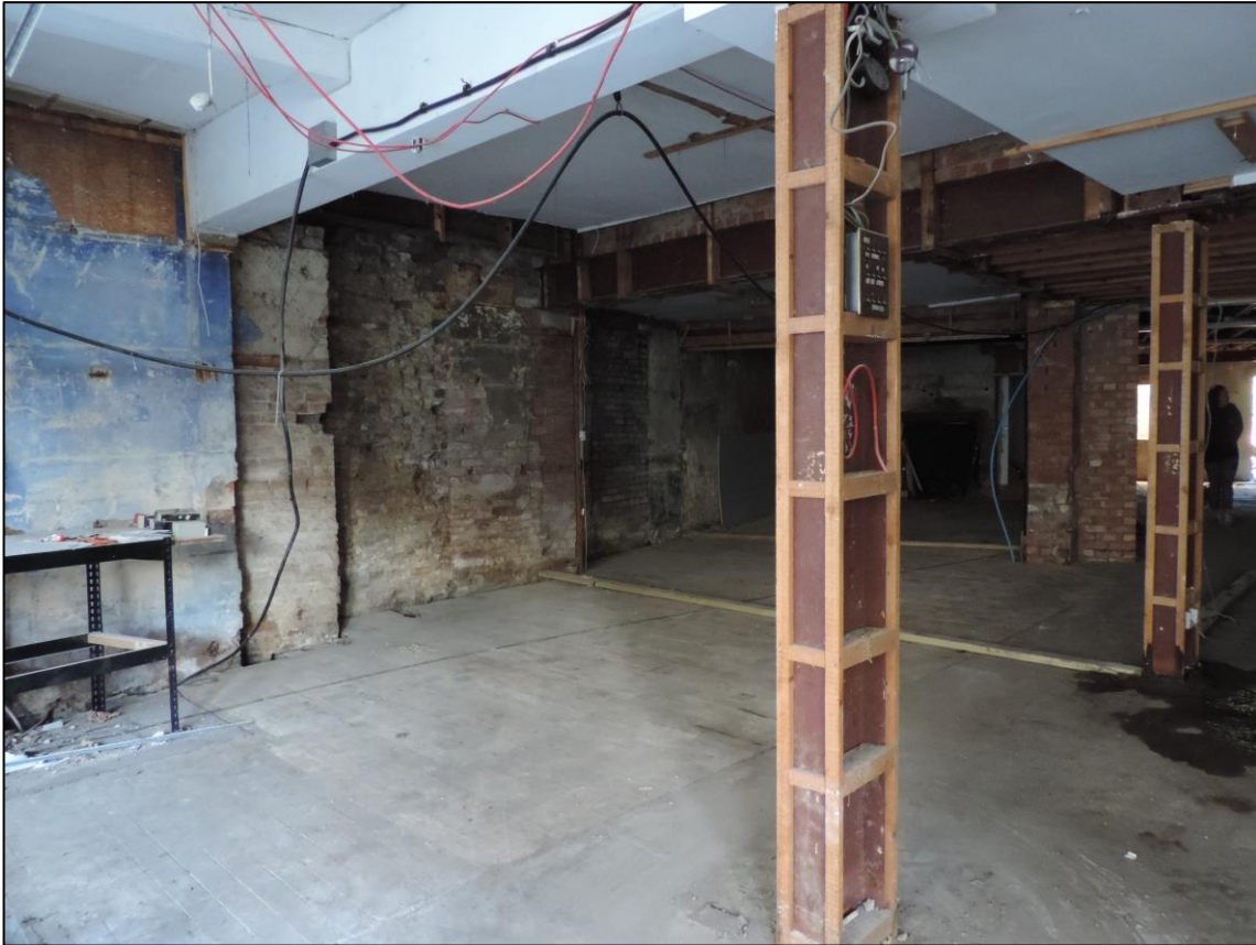
Photo 3 Northwest facing view ground floor no. 20 Church Street showing masonry with brick infilled openings.
