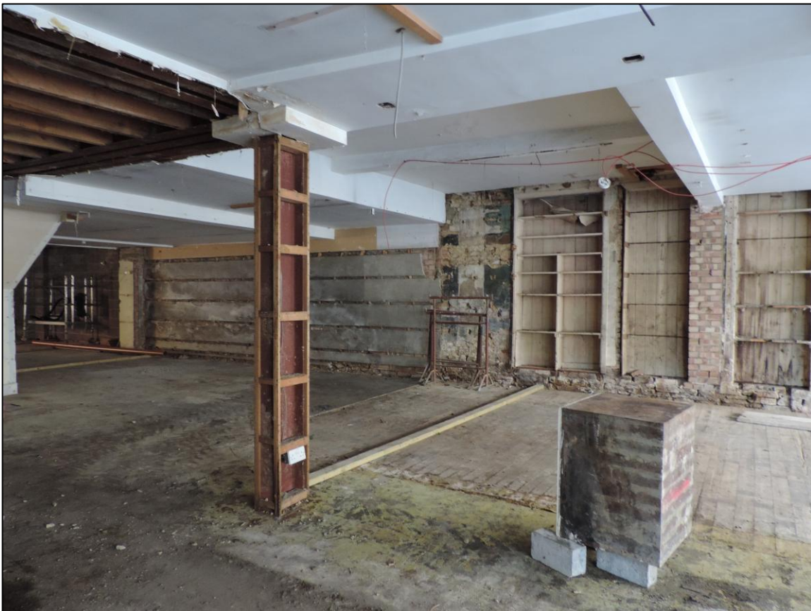
Photo 4 ENE facing view ground floor no. 20 Church Street.
