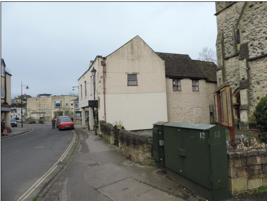
Photo 2 Northwest facing view of the Project Site east elevation from Church Street. Photo taken 27/02/2024.
