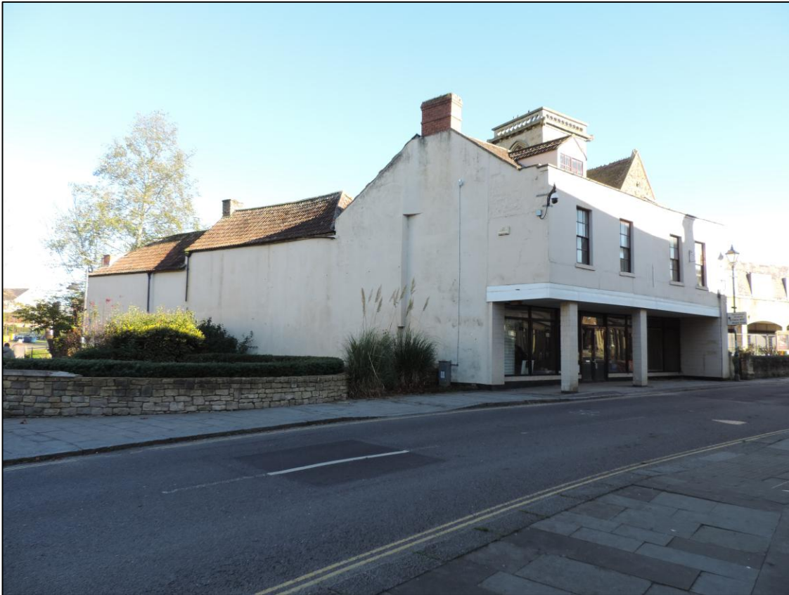
Photo 1 Northeast view of the Project Site with jettied first floor supported on blockwork piers and vacant west elevation. Photo taken 18/11/2025.
