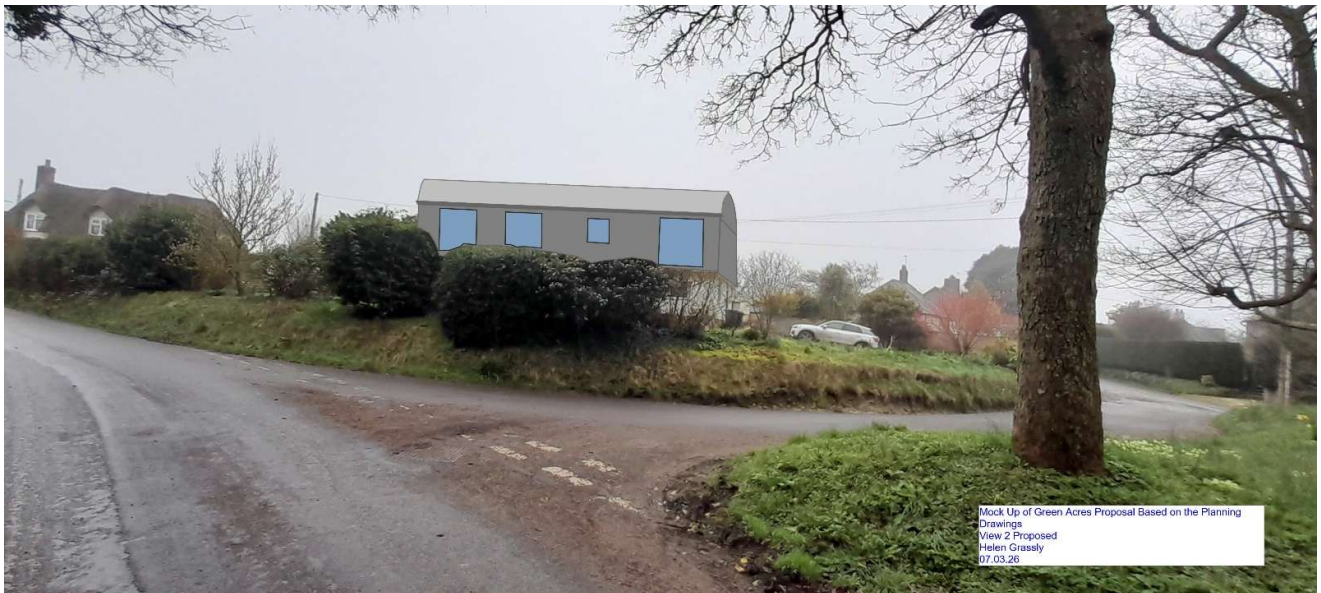
Proposed View 2 at entry to village from South East
