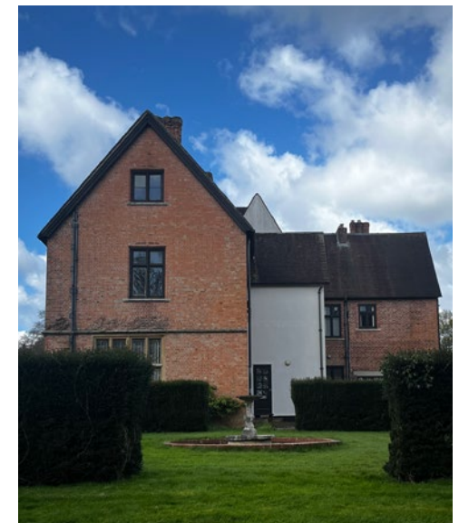
Eastleigh Court East Facade
