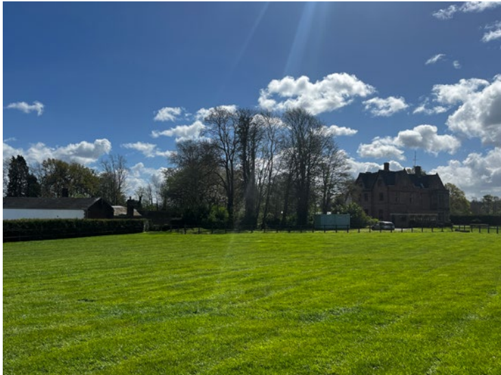
Eastleigh Court & the Former Eastleigh Court Stables approach from north-west
