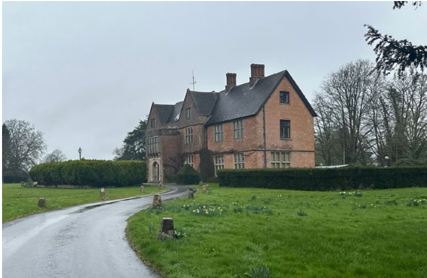
Eastleigh Court approach from south-east
