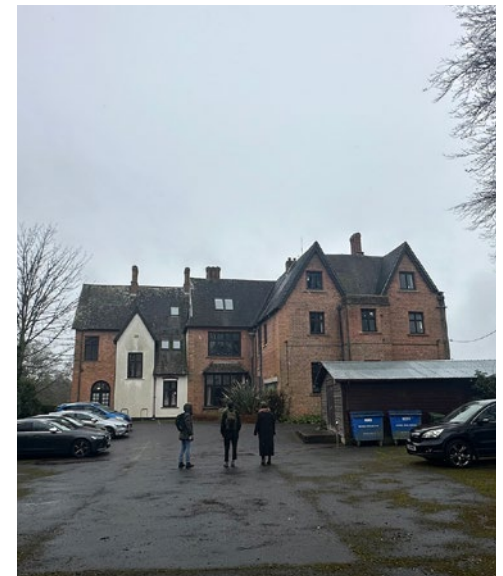
North Facade with 50's rendered extension.
