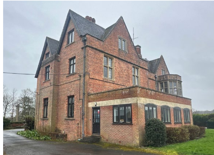
View from north-west with the 1990's extension clearly visible
