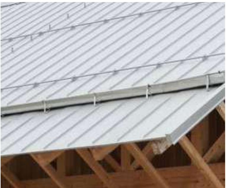
Metal standing seam roof
