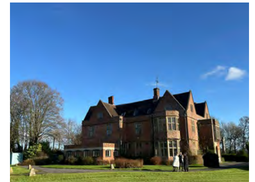
Exterior photo of Eastleigh Court showing proximity of road
