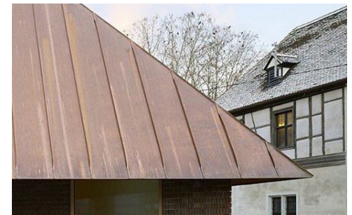
Copper standing seam roof
