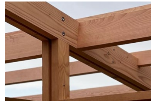
Locally sourced timber frame
