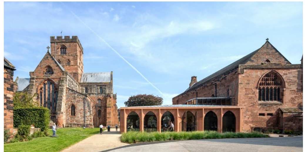
Contemporary stone extension sitting harmoniously with historic building. Carlisle Cathedral by Fielden Fowles
