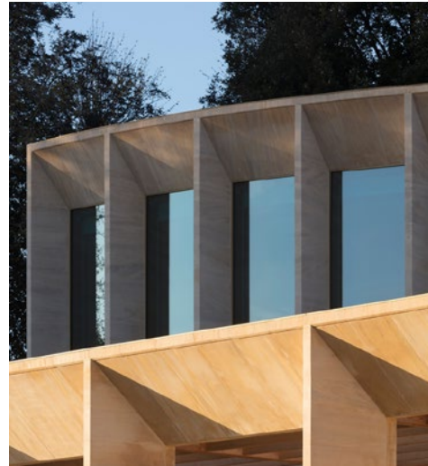
Chamfered stone mullions by Niall McLaughlin Architects
