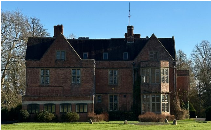
West elevation of Eastleigh Court
