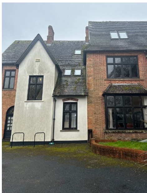
60's rendered stairwell to rear
