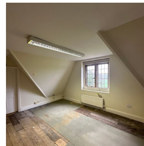
2nd floor with original windows and floorboards but lacking heritage detail
