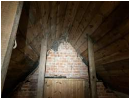
Photograph 19: Void 3 looking eastward
