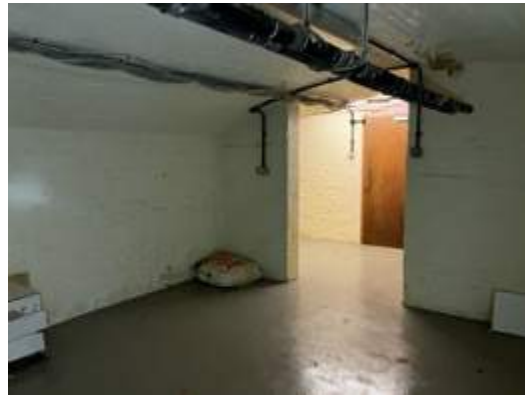
Photograph 20: Basement accessed from inside
