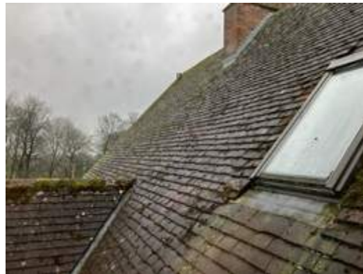
Photograph 16: View of roof with PRFs
