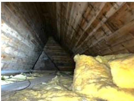
Photograph 17: Void 1 looking westward
