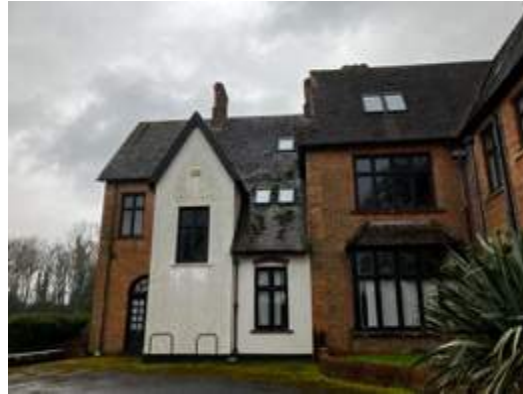
Photograph 14: Northeast elevation of Eastleigh Court
