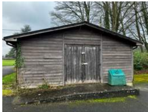
Photograph 22: Eastern elevation of the Garage
