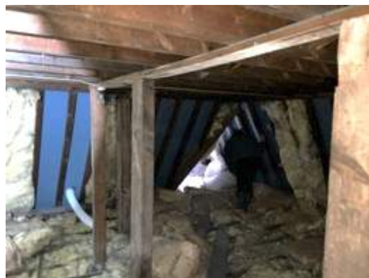
Photograph 18: Void 2 looking northward
