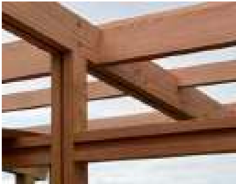
Local Timber Frame
