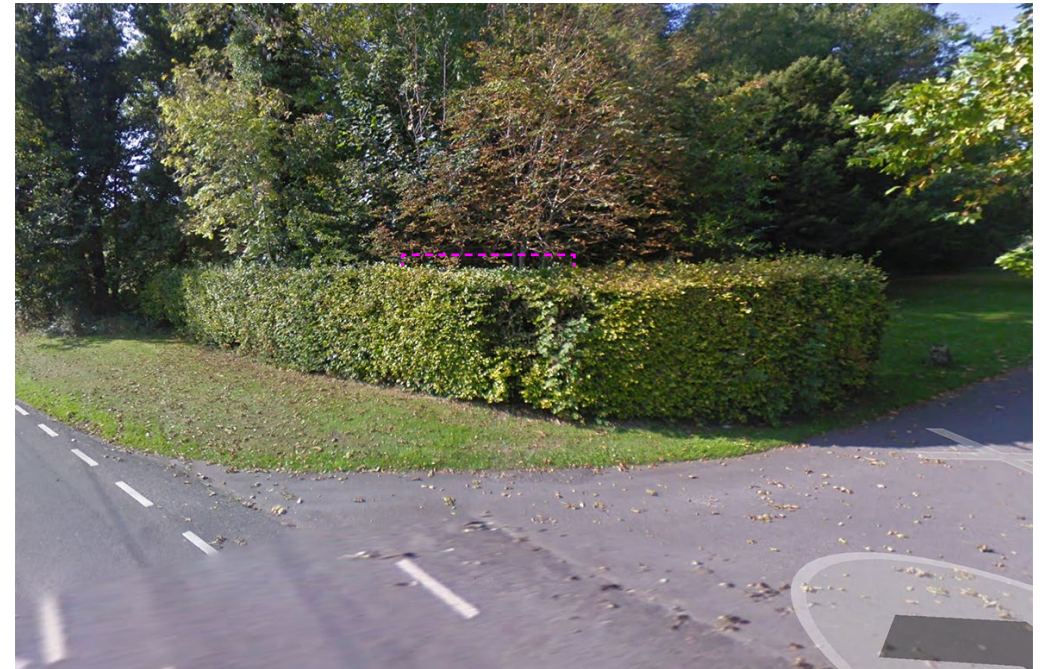
Photo from Bishopstrow Road looking south with location of substation indicated in pink
