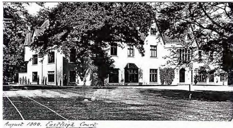
Figure 5: Photocopy of a photograph showing the principal (south) front of Eastleigh Court in 1888 with western extension of a similar scale to that on the east (from bay window and to the left).
