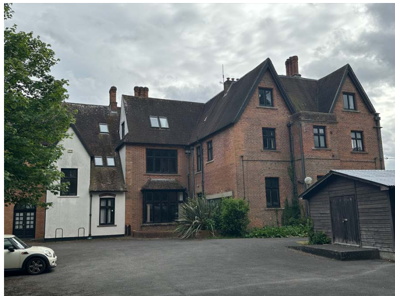
Figure 22: northern elevation of Eastleigh Court with 'modern' stair to the left and concrete lintel for the former garage doors in the centre.
