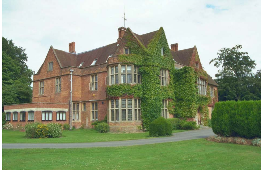
Figure 1: Eastleigh Court as photographed in 2000 as part of the Images of England project (Historic England; IoE01/02471/06)
