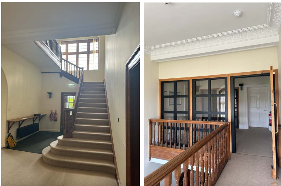
Figures 18 & 19: Staircase (July 2024)
