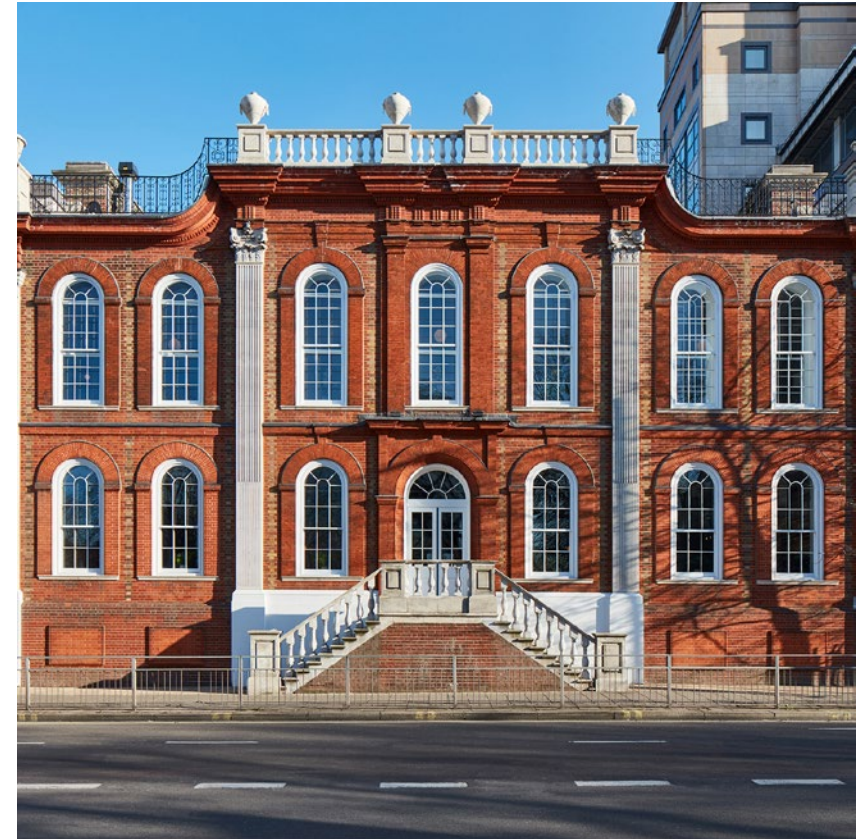
Kindred Hammersmith - First floor multi-functional space
