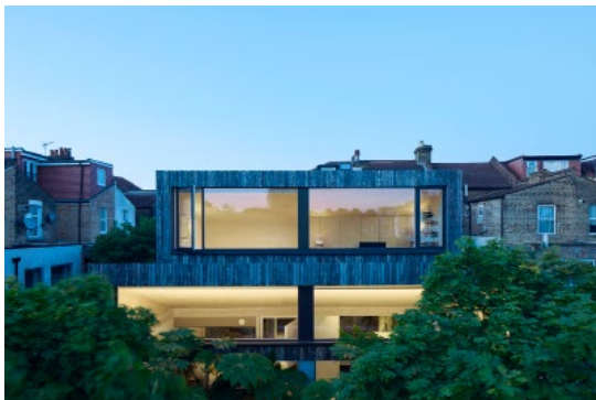
2 new houses, east London
