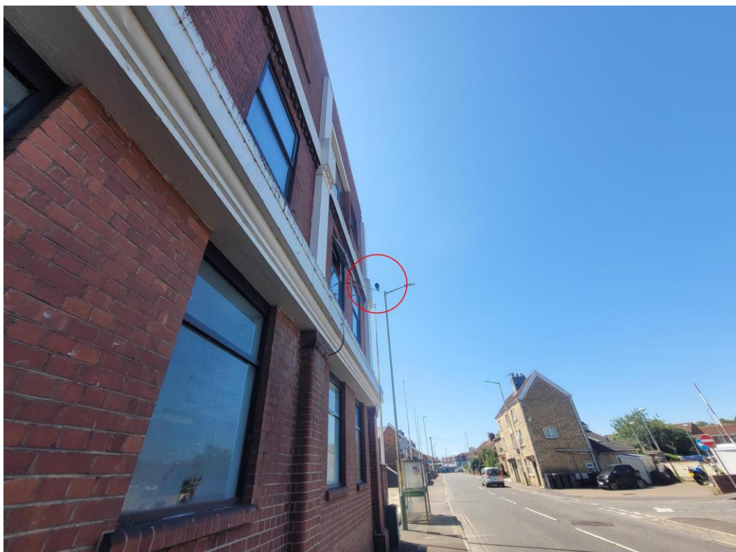
Figure 6: A photo of MP1 taken from A3102 looking west
