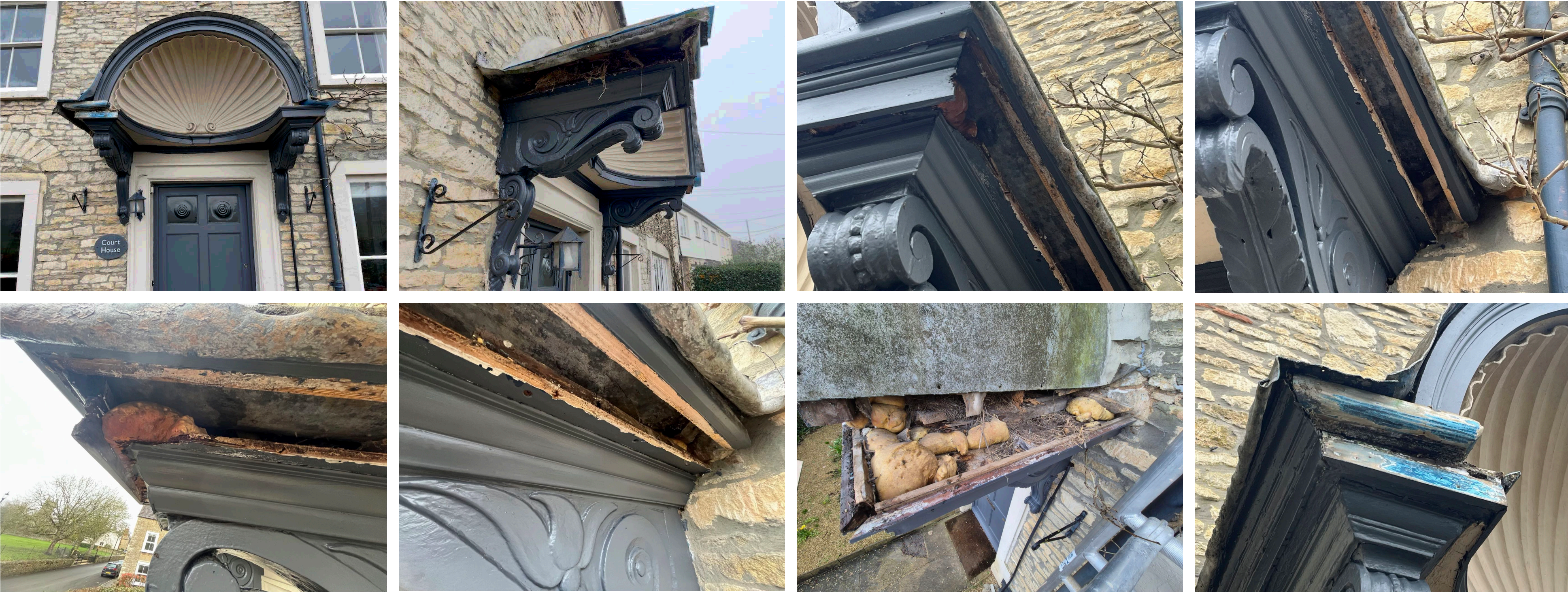
PORCH. EXISTING PHOTOGRAPHS
