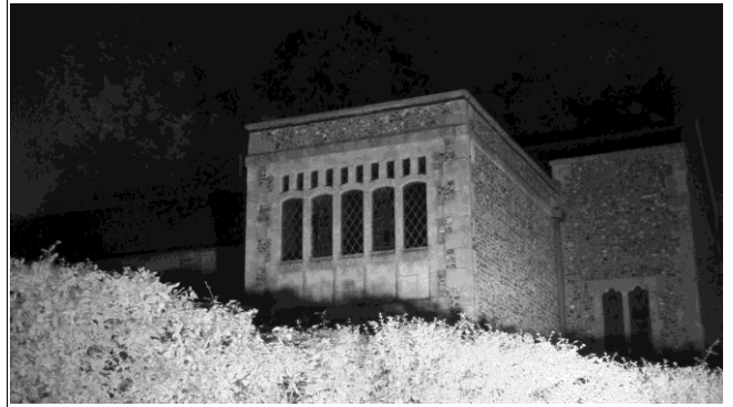
Photograph 24. IR still image of the south eastern elevation (Surveyor 4), during the third dusk survey on 14 th July 2025
