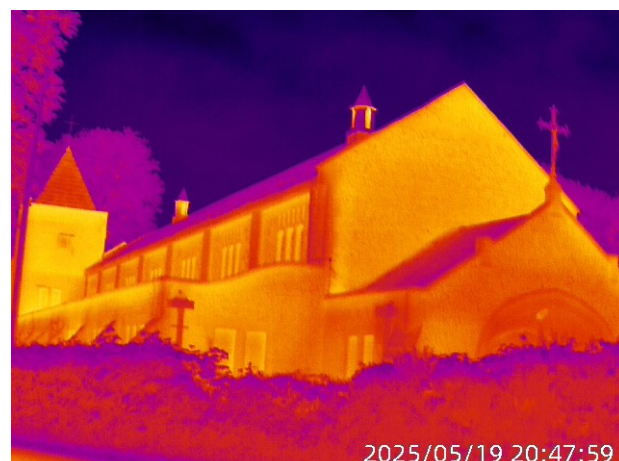
Photograph 14. Thermal image of the north western elevation (Surveyor 2), during the first dusk survey on 20th May 2025
