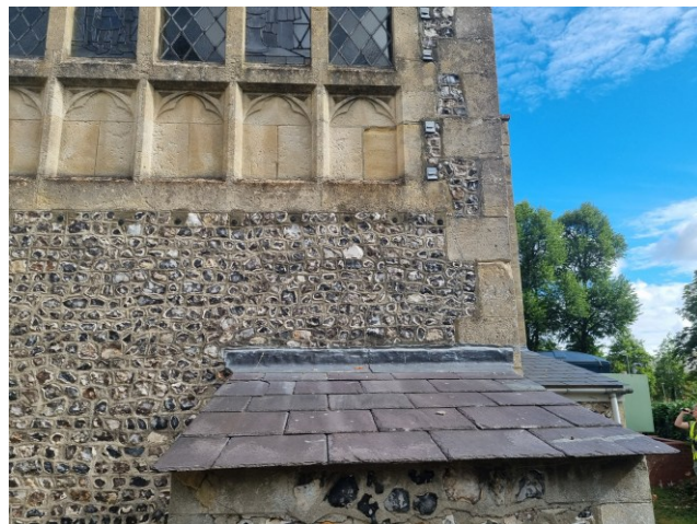
Photograph 3. Location of the pump room on the eastern end of the southern elevation of the church
