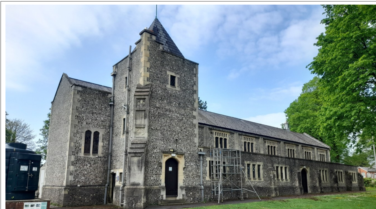
Photograph 1. General view of the northern elevation of the church and tower.
