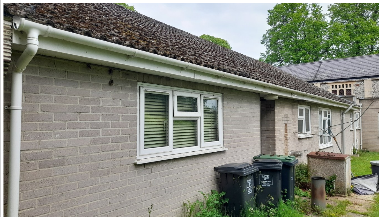
Photograph 2. Eastern elevation of the adjoining bungalow (presbytery)
