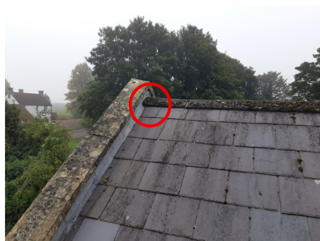
Photograph 8. North side of the raised eastern ridge tile on the main roof.
