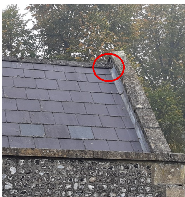
Photograph 9. South side of the raised eastern ridge tile on the main roof.
