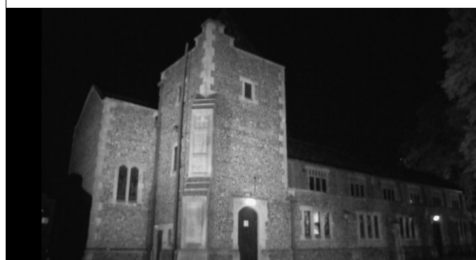
Photograph 16. IR still image of north eastern elevation (Surveyor 3), during the second dusk survey on 16th June 2025
