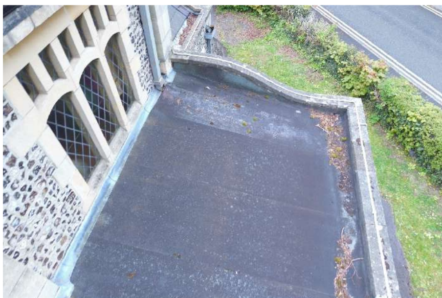
Figure 22 – Existing Mineral Felt Aisle Roofs
