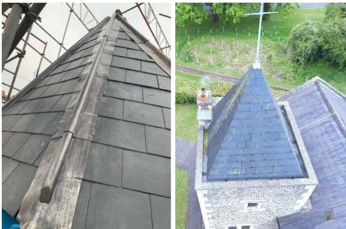
Figure 20 & 21 – Example of rolled leaded hip(left), and existing fibre cement tiles and concrete hip to Nave (right)
