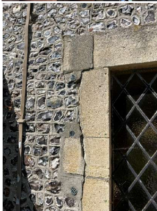
Figure 16, 17, 18, 19 – Photographs of example damaged stonework, and internal water ingress.
