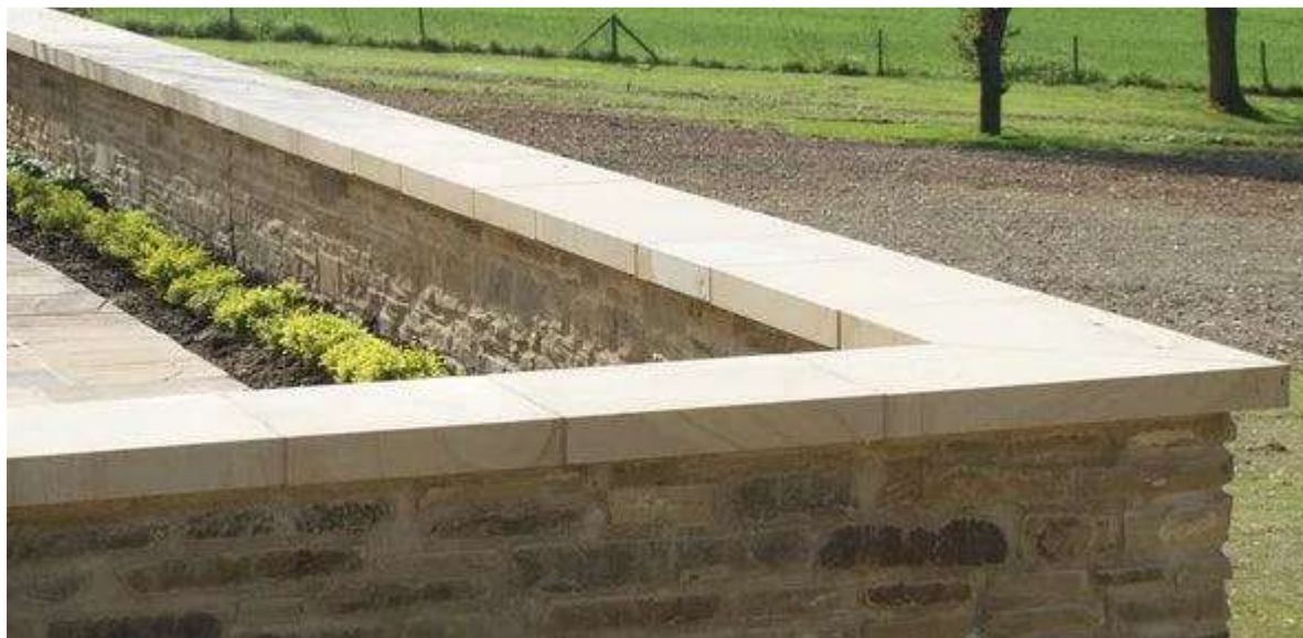
Figure 36 – Bath Stone Capping Example for retaining wall
