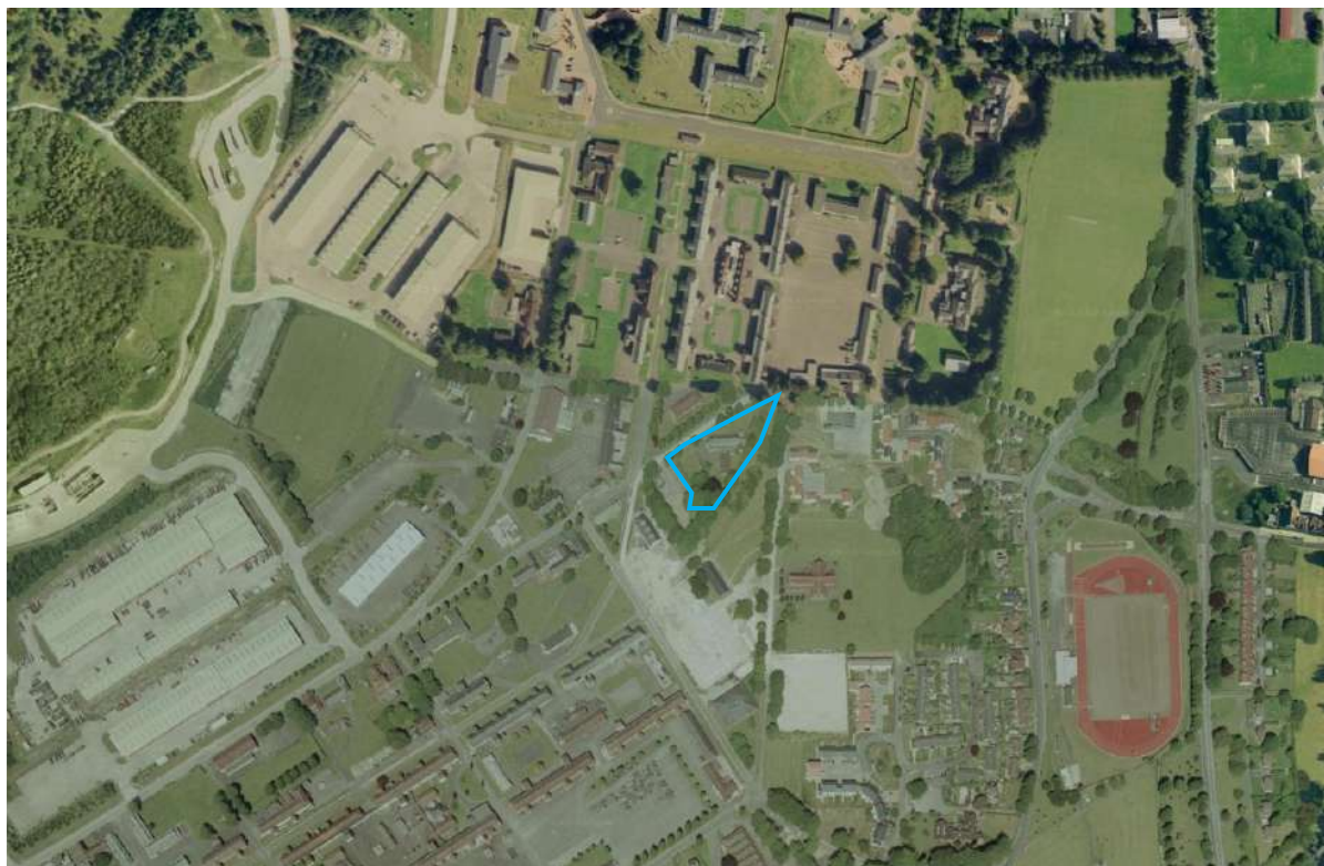
Figure 7 - 1999 Aerial – The more recent aerial photography, shows the beginning of the consolidation of smaller buildings into larger structures to meet modern requirements.
