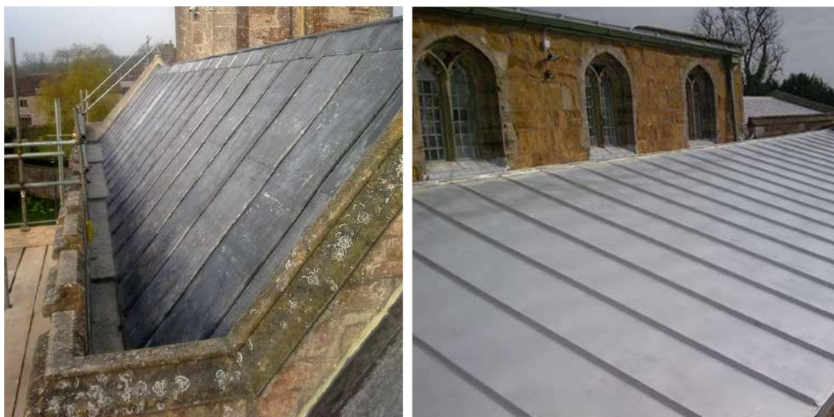
Figure 27 & 28 – Example of lead standing seam on church (left), Example of zinc/steel standing seam (right)
