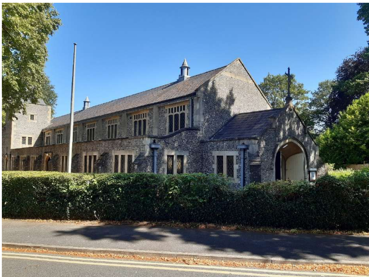
Figure 11 - View of St Patrick's Garrison Church from St Patrick's Avenue, looking East
