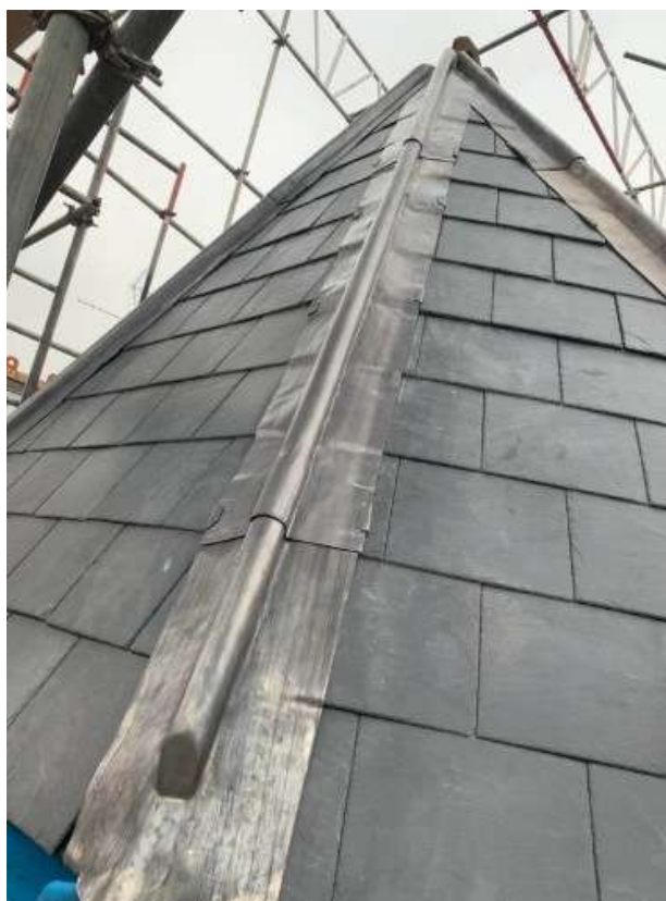
Figure 13 & 14– Example of rolled leaded hips
