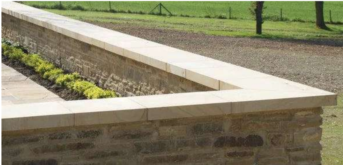
Figure 31 – Bath Stone Capping Example for retaining wall
