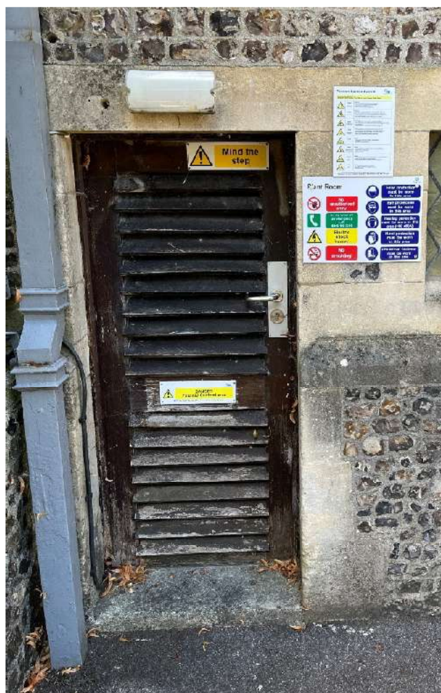
Figure 18 & 19 – Rotten plant door and more robust PPC aluminium door
