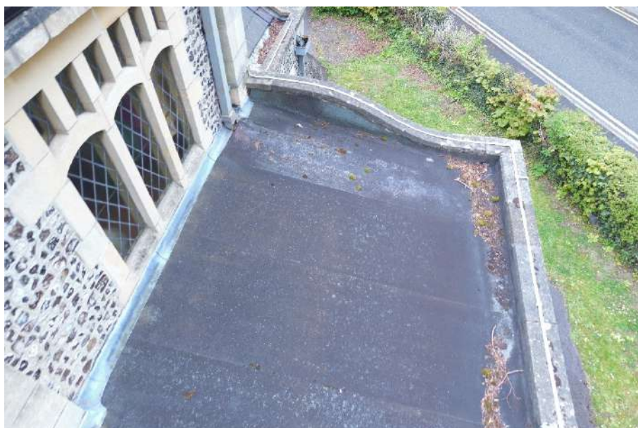
Figure 15 – Existing Mineral Felt Aisle Roofs
