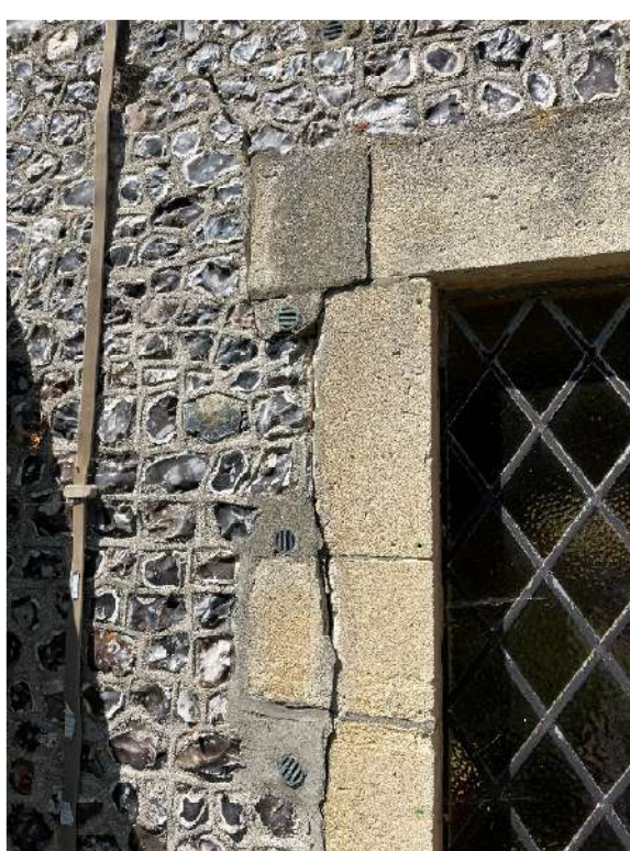
Figure 3, 4, 5 & 6 – Photographs of example damaged stonework, and internal water ingress.
