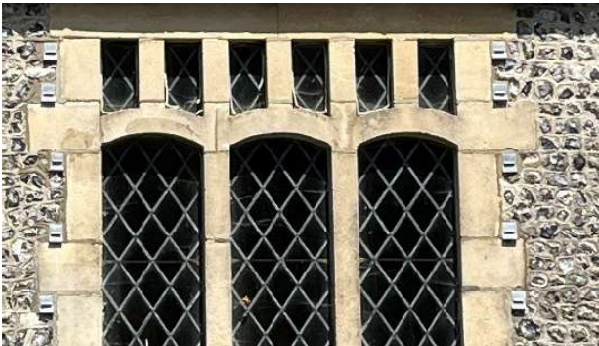
Figure 17 – Example of knapen vent caps installed to other areas of the building
