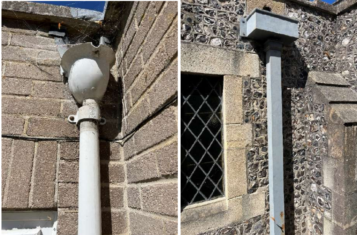
Figure 25 & 26 – Existing uPVC rainwater goods (left) to be replaced with cast iron to match existing profiles (right)
