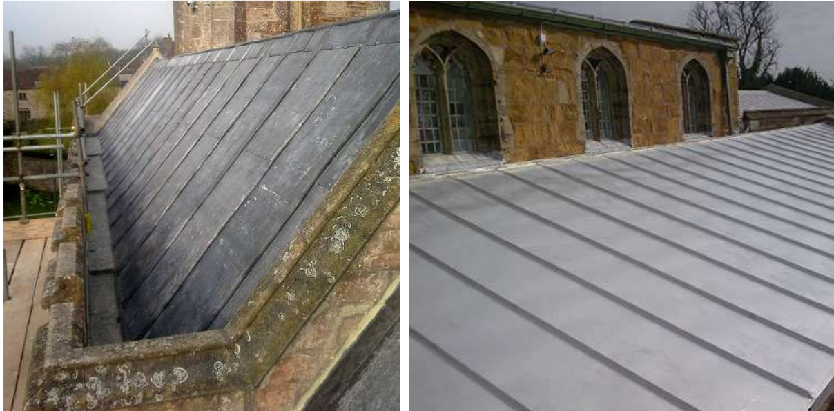
Figure 20 & 21 – Example of lead standing seam on church (left), Example of zinc/steel standing seam (right)
