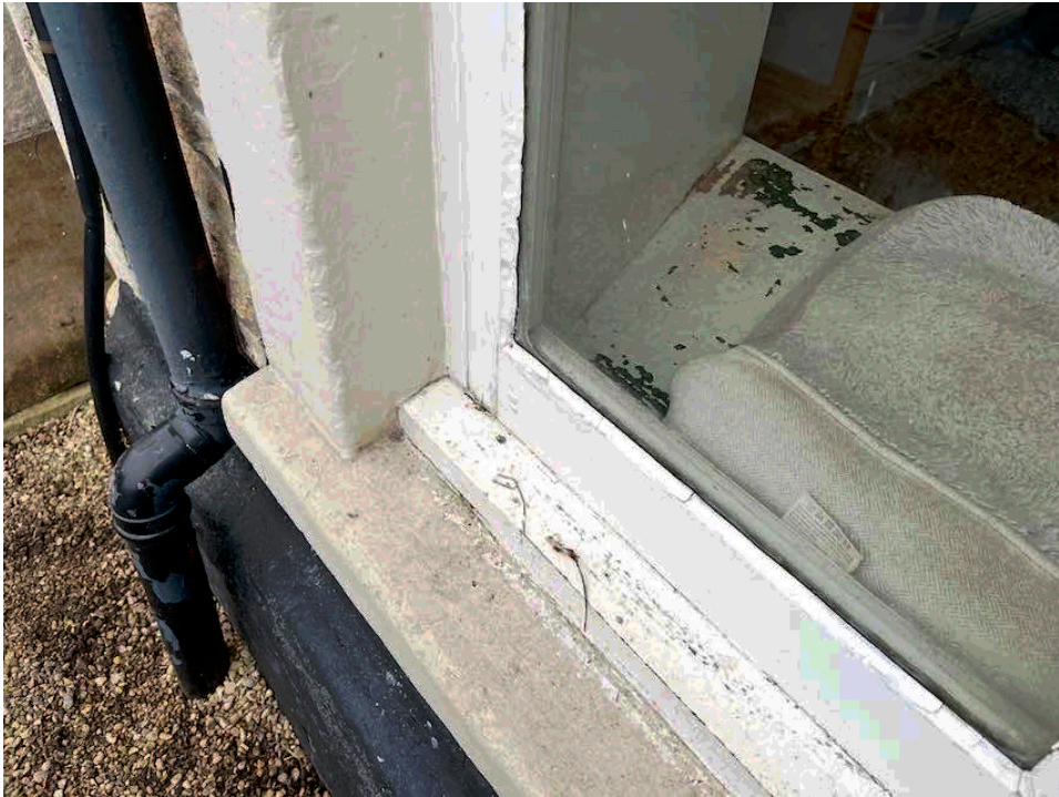
EXISTING WINDOW EXAMPLE ON NORTH AND EAST ELEVATIONS
