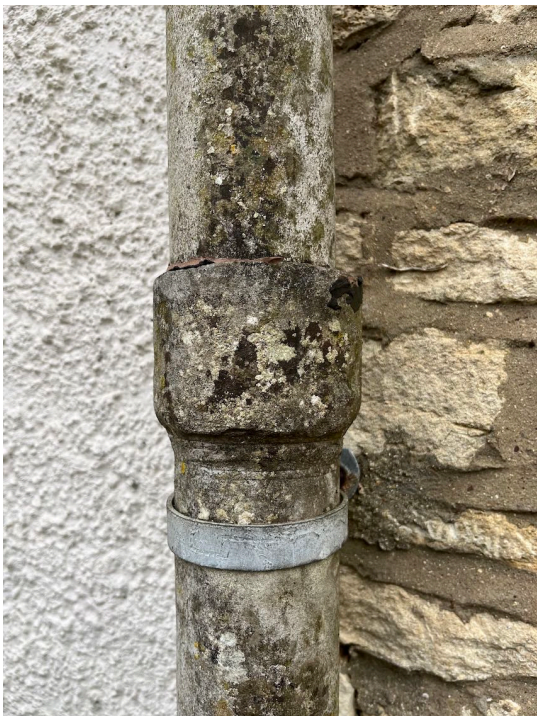
EXISTING ASBESTOS DOWNPIPE
