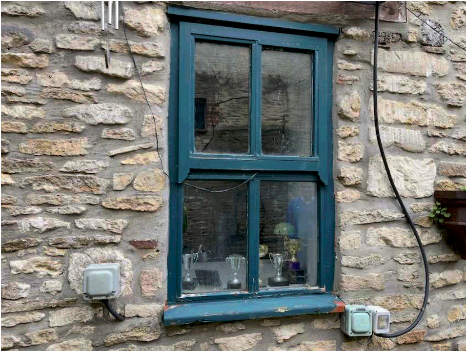
EXISTING WINDOW EXAMPLE ON SOUTH AND WEST ELEVATIONS
