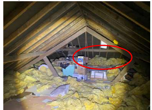
Plate 21: Build up of insulation at adjoining side porch
