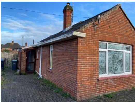
Plate 6: Main building – B1
