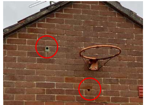
Plate 25: Roof felt tear
