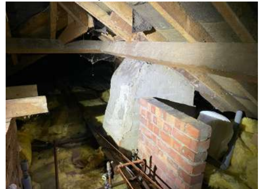
Plate 21: Build up of insulation at adjoining side porch
