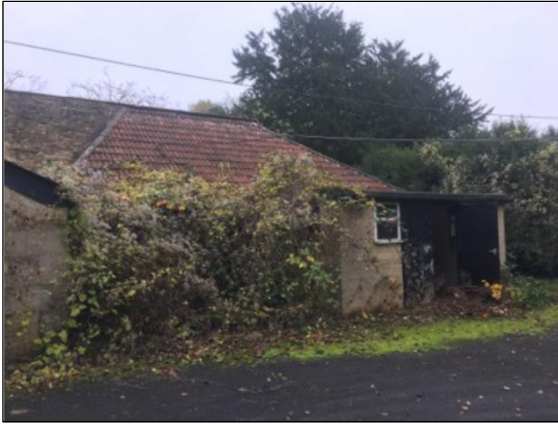
Photograph 3: Western elevations of Building 3
