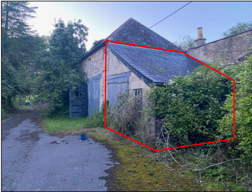
Photograph 11: Lean-to on Building 3 containing lesser horseshoe satellite roost
