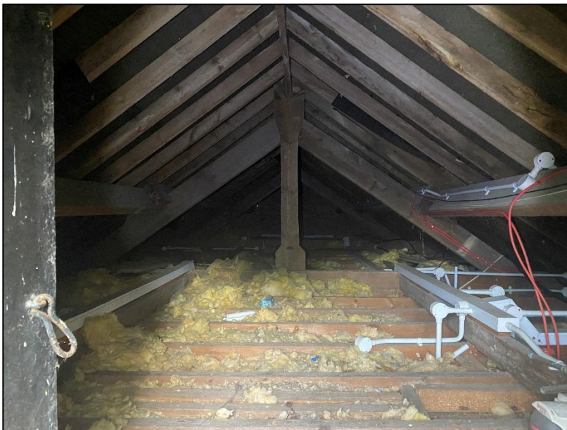
Photograph 4: Loft space above Building 4
