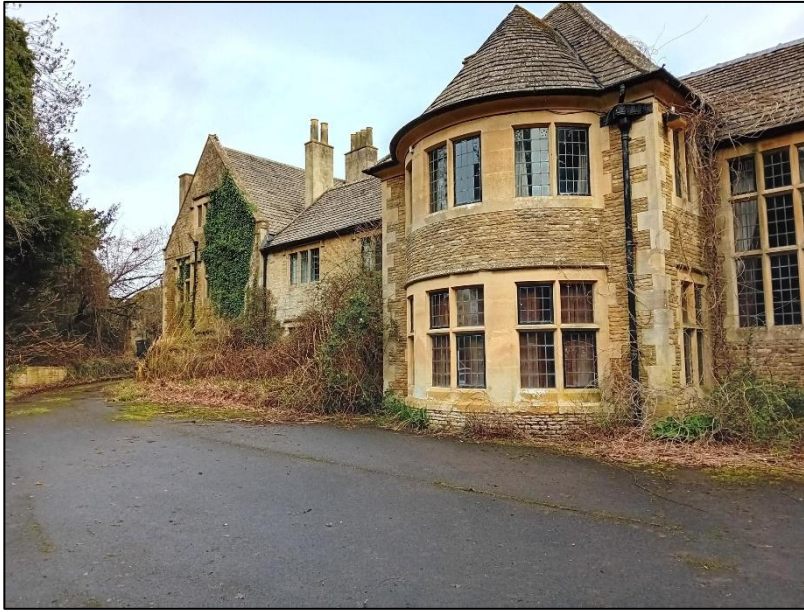
Photograph 1: Western elevation of Building 1 (Pockeridge House)
