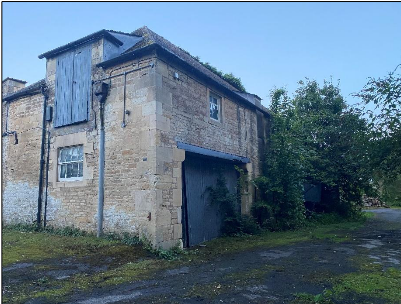
Photograph 2: North and western elevations of Building 2
