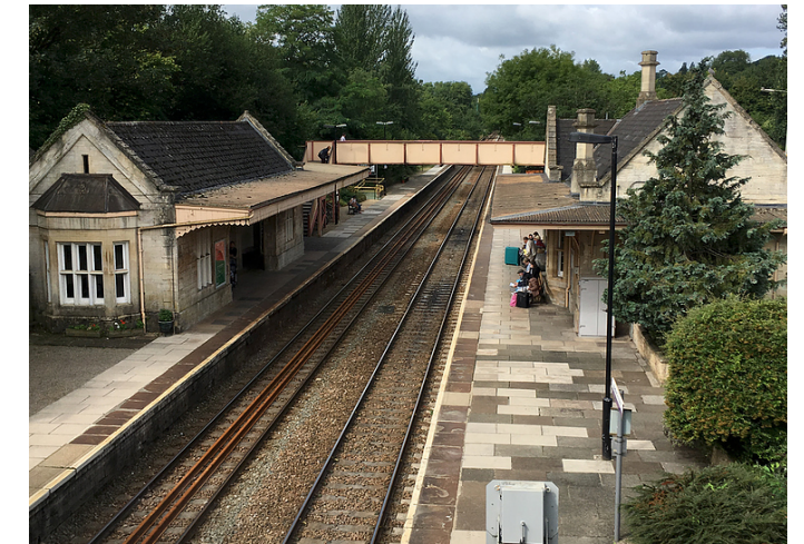
Photograph of the two platforms linked by the footbridge
