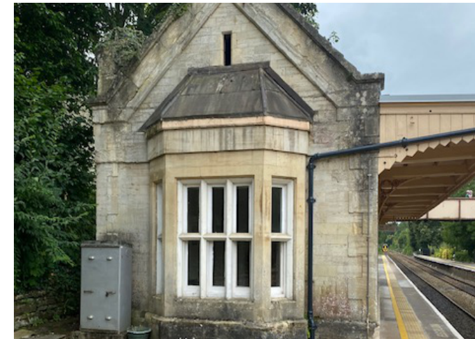
East Elevation of South Platform Building
