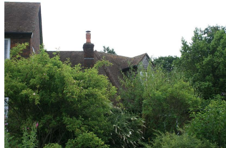
Photo 9: South elevation of the annexe (B1).
