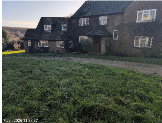
Photo 40: Northern elevation of the house ('B1').
