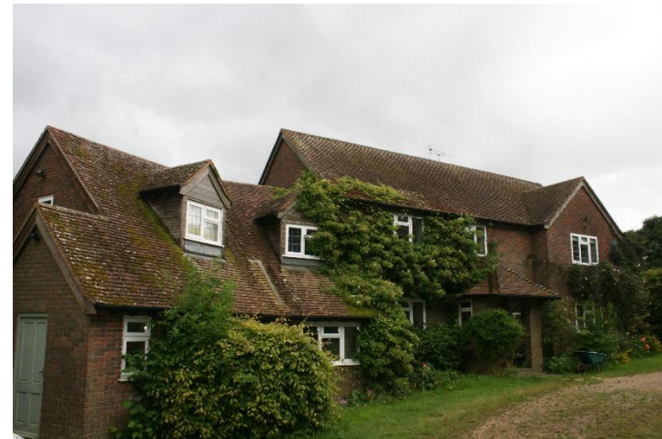
Photo 12: Northeast view of the house (B1).
