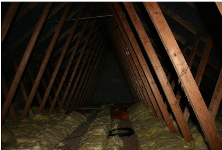
Photo 2: Inside the loft void.
