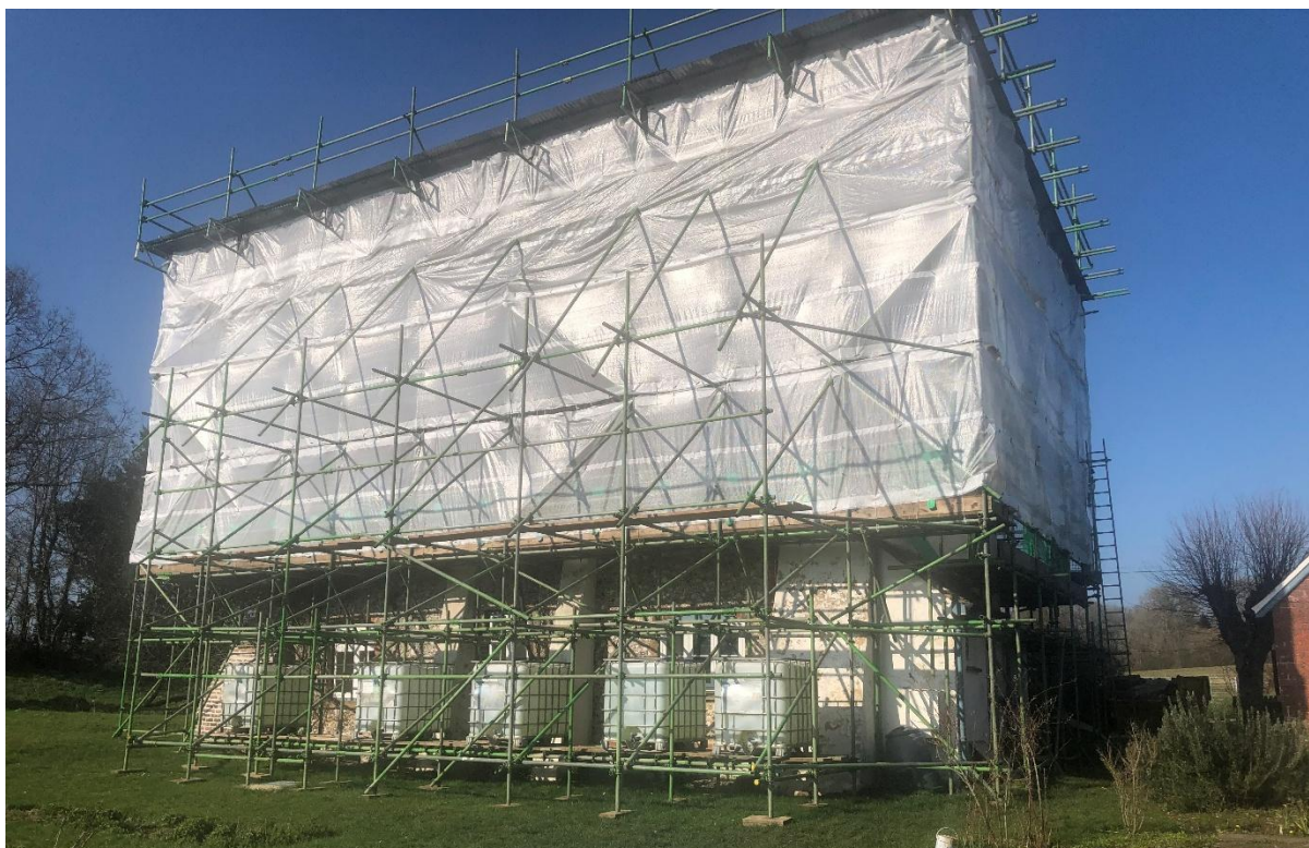
Figure 6 – Current photo of the property with ‘roofed over scaffolding’ in place
