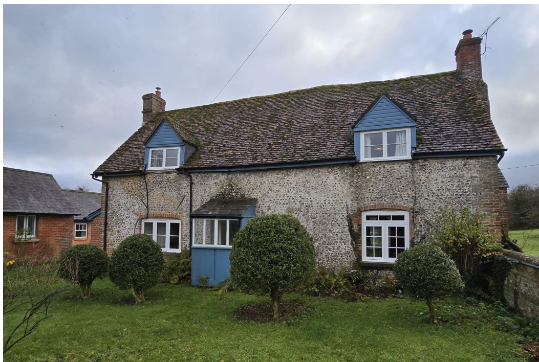
Figure 4 – Front elevation of Jolly's Farmhouse prior to roof repair
