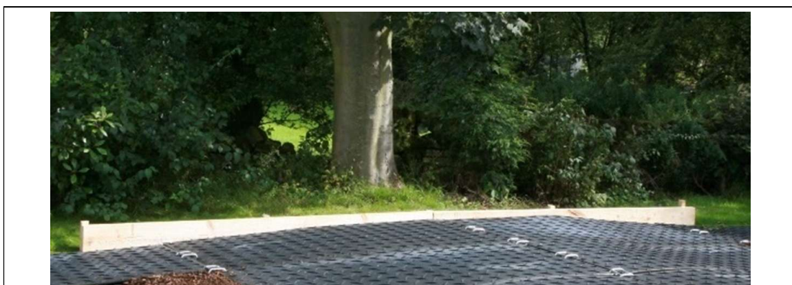
Figure 4: Example of proprietary, inter-linked ground protection boards used to protect RPAs.
