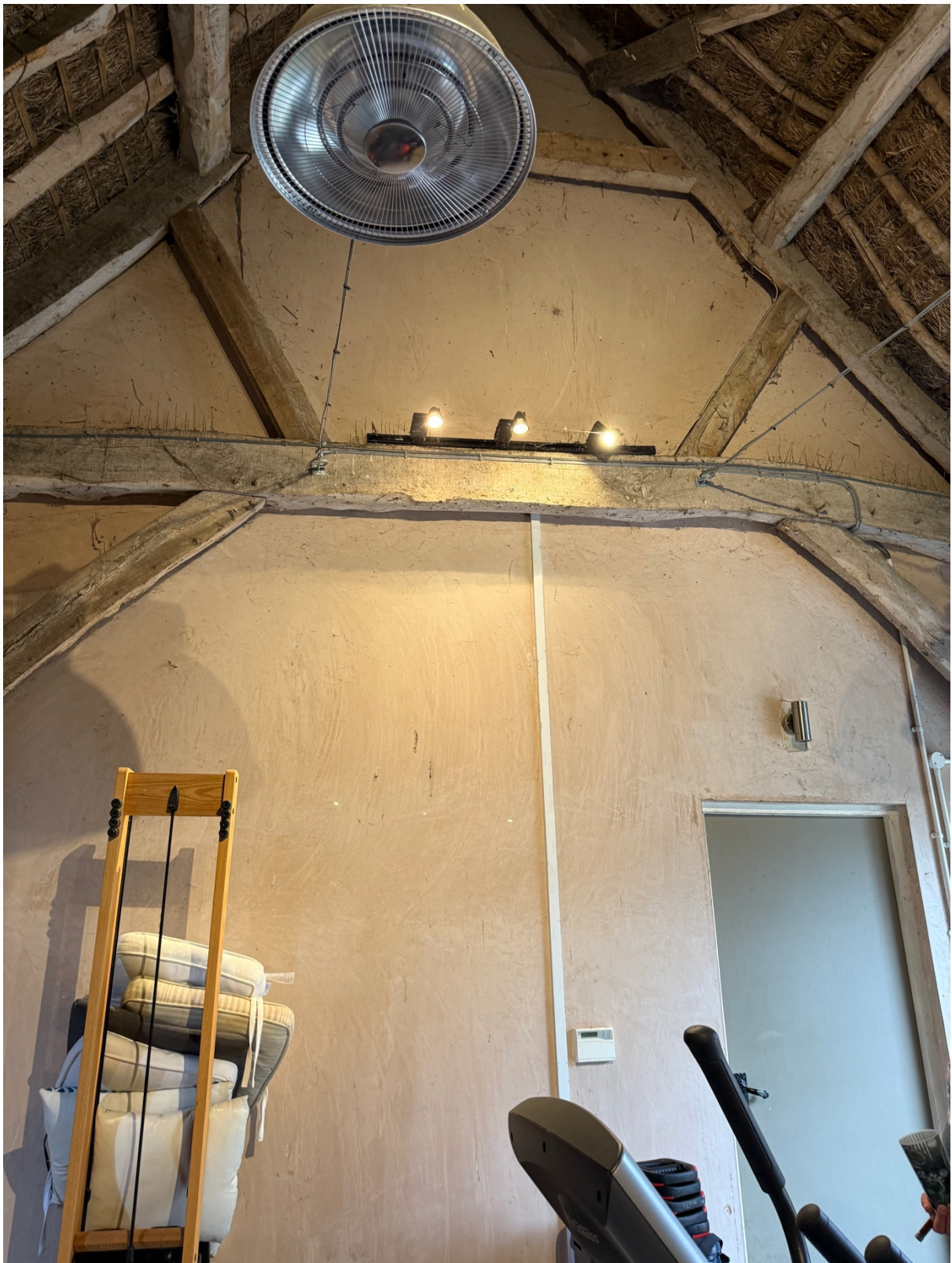
Existing structure and inserts retained
