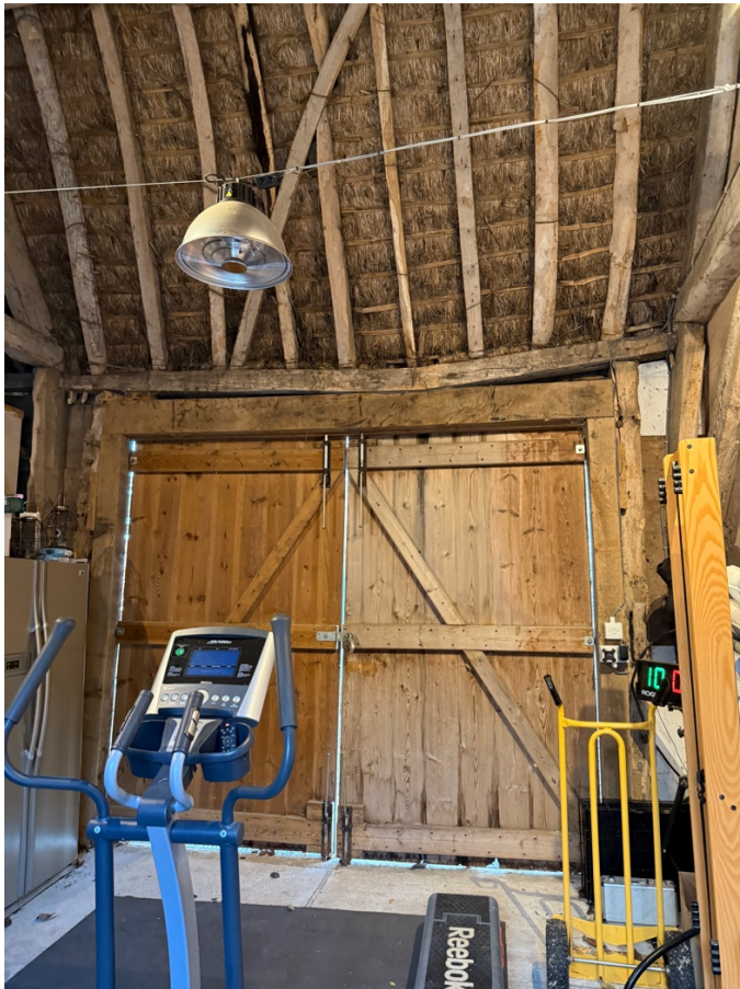
Barn Doors retained; new glazed doors mounted on Door frame
