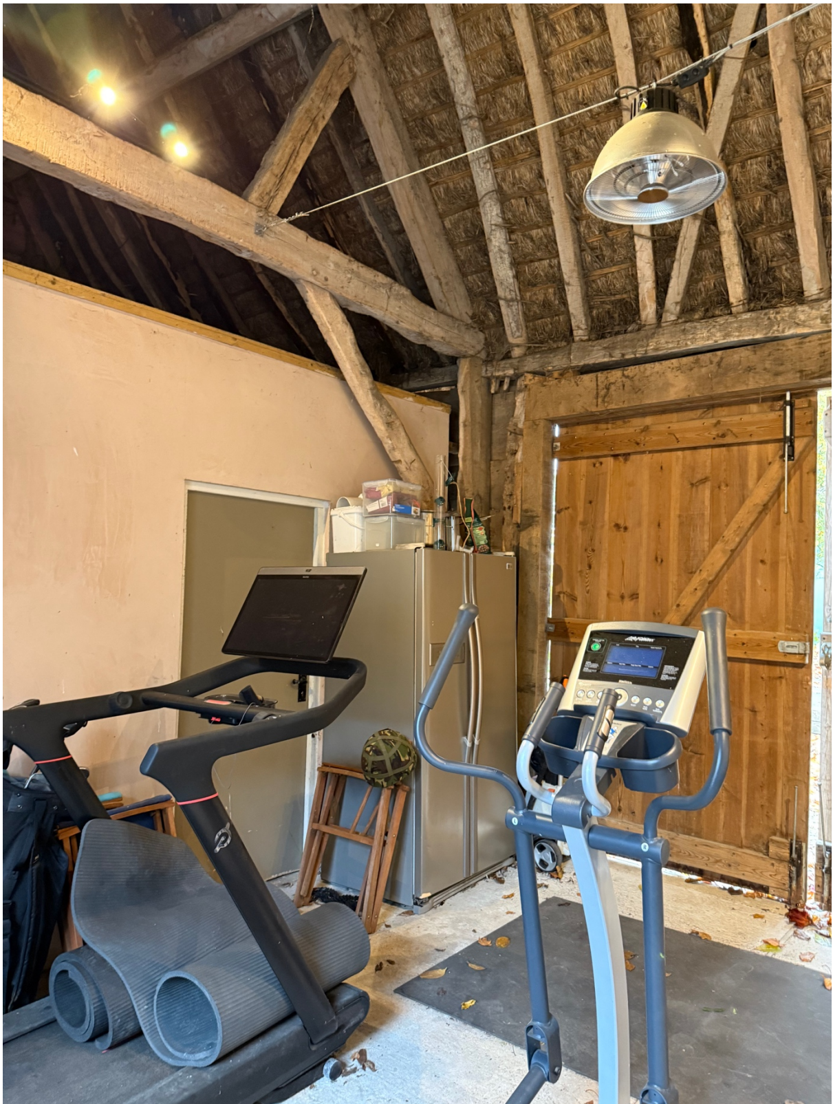
Inserted Wall removed retaining mezzanine floor.
