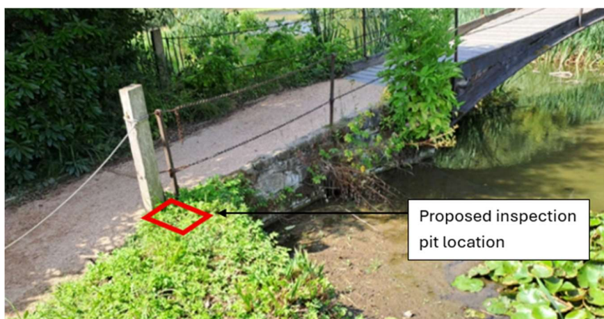
Figure 1 – Inspection pit location
